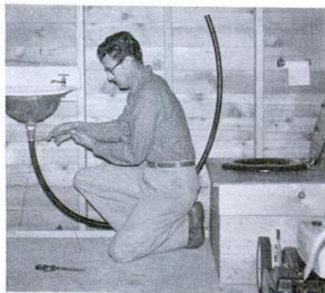
PLASTIC TUBING is fitted to washbasin drain and extended along base of wall to the drum, providing an additional water supply for flushing of the toilet
