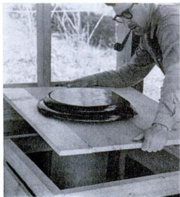
BOX BUILT OVER DRUM supports conventional toilet seat, under which the flanged top of the galvanized pipe is attached to a 2-ft.-square board platform
