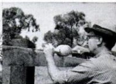
Trim fence posts
