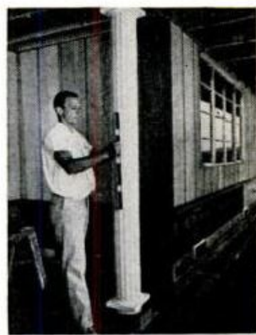
4: Locate column, using 2x4 prop. Check work with level
