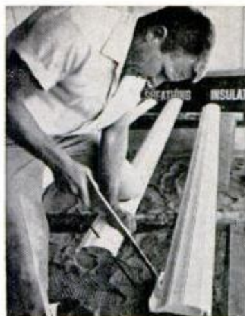
1: Cut column staves to length, using hand or power saw
