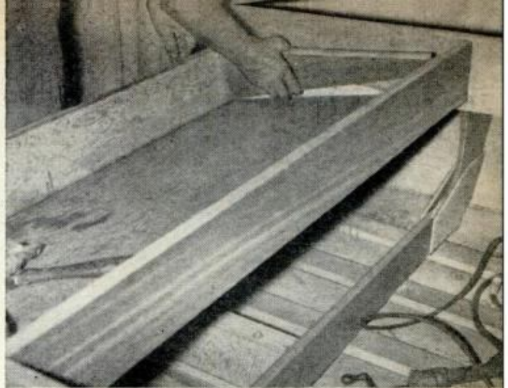
MOTOR-WELL BOTTOM fastens to bottom edge of well beam and to side blocking, shown here being fitted
