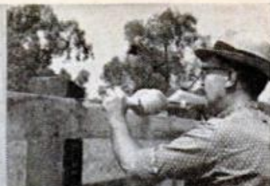
Trim fence posts
