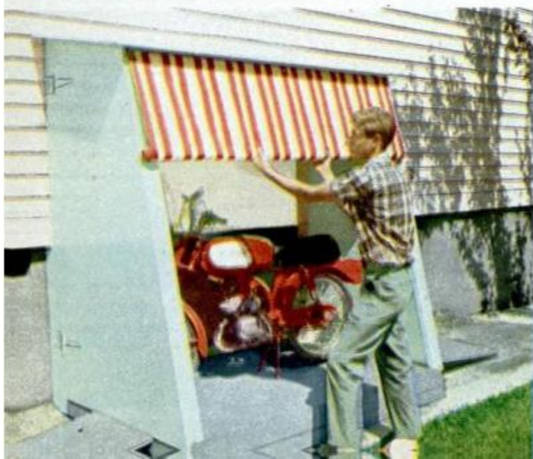
CANVAS LEAN-TO. Designed to attach to the side of a garage or house, this walk-in lean-to version, with its drop-curtain front, opens wide to give complete access. Canvas flap buttons to facing strips on doors
