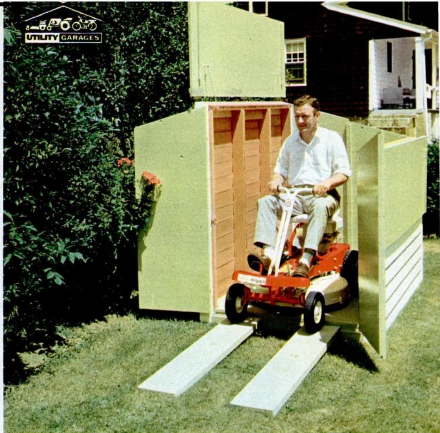
DRIVE-THROUGH SHELTER. You can drive in as well as drive right out of this little garage since it has doors at both ends. Roof sections, which lap one another, fold up and over, one being held vertical by long hooks and screw eyes. While twin ramps merely rest level with floor, they could be hinged to fold up inside unit
