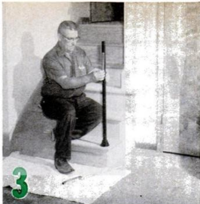
PLUMB THE NEWEL POST with a level after inserting it in the floor flange. When vertical, anchor it by tightening the slotted setscrews in the flange
