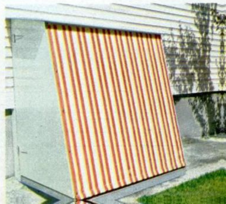
CANVAS LEAN-TO. Designed to attach to the side of a garage or house, this walk-in lean-to version, with its drop-curtain front, opens wide to give complete access. Canvas flap buttons to facing strips on doors
