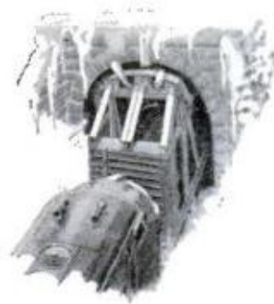
BULKHEAD FLATCARS normally transport pulpwood or wallboard. But some Clinchfield R.R. jobs run interference for auto transporter cars in the winter, clearing away destructive ice from roofs of tunnels
