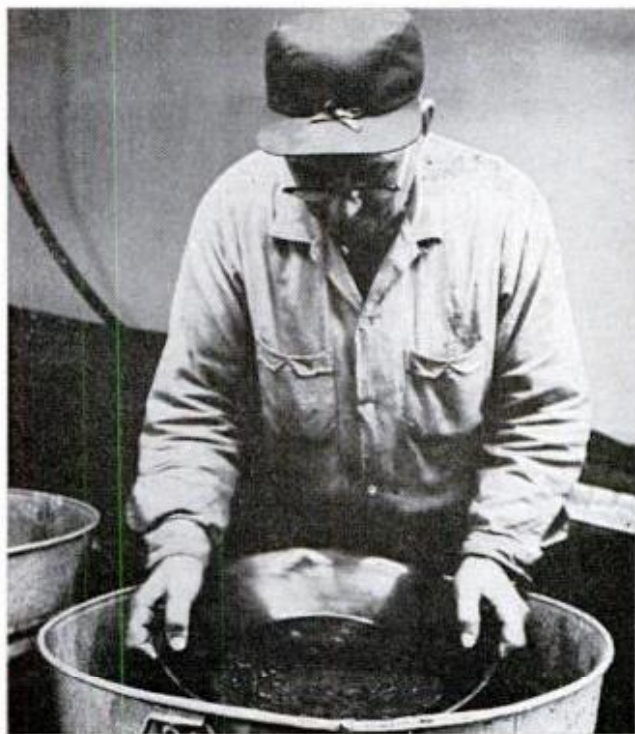
TESTING FOR COLOR , a prospector pans the gravel and sand taken from a test coring. This old method is still the most effective for finding samples
