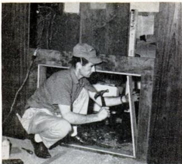
OPENING FOR TV SET is cut beneath screen with saber saw, and \frac{3}{4} x4-in. solid teak strips are mounted with glue and finishing nails so front edge protrudes \frac{1}{4} in.
