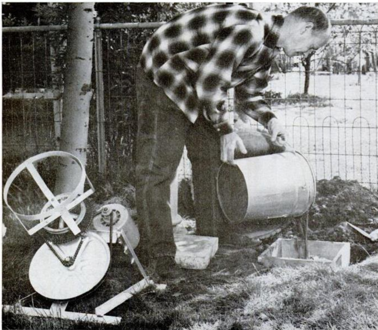
RIGHT FROM THE MIXER into the form for a birdbath footing goes this batch of home-brewed concrete
