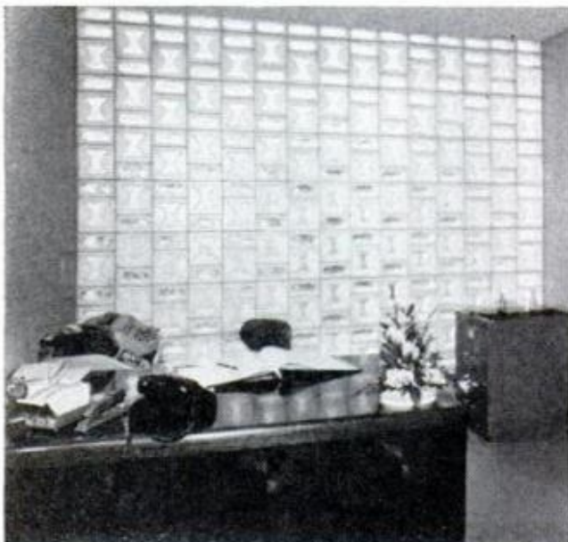
TRANSLUCENT GLASS-BLOCK WALL features hour-glass and oval pattern. Steel reinforcing strips were inserted in mortar joints to add strength to the wall
