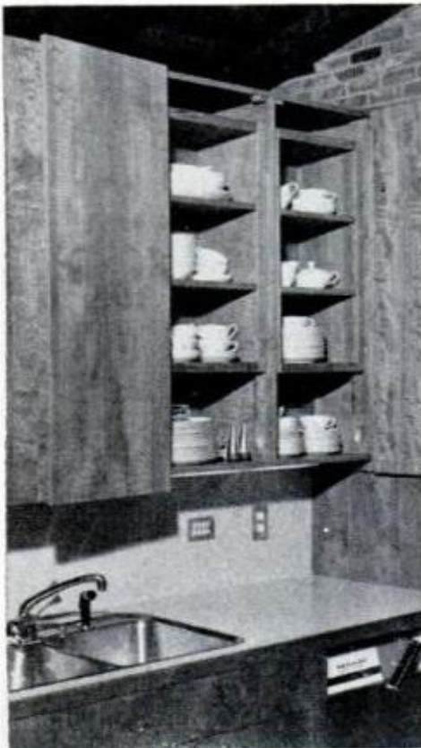
CABINETS IN POSITION (above) make a neat installation. The 1\frac{1}{2} -in. cupboard frame conceals most of the brackets. Even a short person has no trouble in reaching the top shelf when the cupboard is swung down (right)
