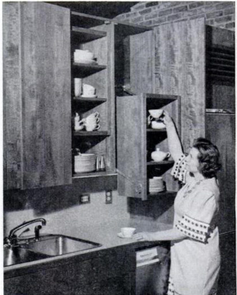
CABINETS IN POSITION (above) make a neat installation. The 1\frac{1}{2} -in. cupboard frame conceals most of the brackets. Even a short person has no trouble in reaching the top shelf when the cupboard is swung down (right)
