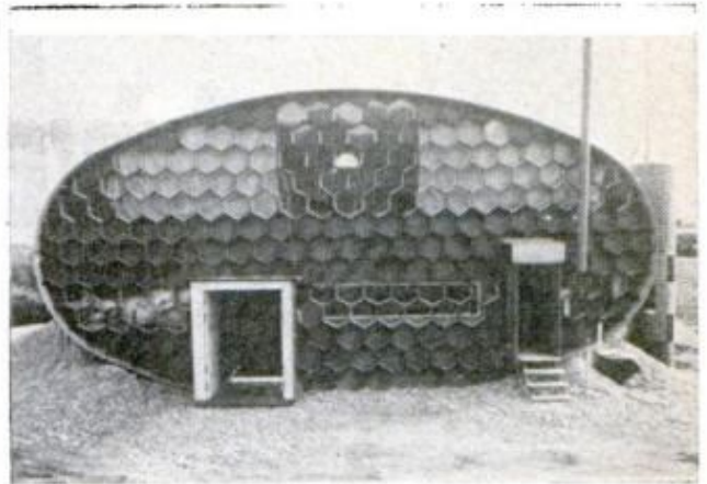
Corrugated-metal house , made of 114 steel plates formed into an oval shape, has been constructed in Tokyo. The unusual two-level dwelling has no foundation but rests on a bed of sand, because of the hazard of earthquakes.
