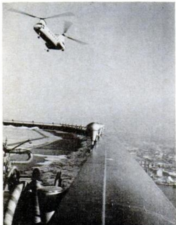
Helicopter landings on top of the PanAm building in New York City are made safer by a system of louvered aluminum vanes installed around the perimeter of the roof (photo, left). The vanes control air flow over the roof by catching turbulent currents and releasing them in a smooth flow. The system will allow safe operations in steady winds up to 60 mph and gusty winds up to 50 mph. Center building in the wind-tunnel study (above) has vanes that smooth out air currents.
