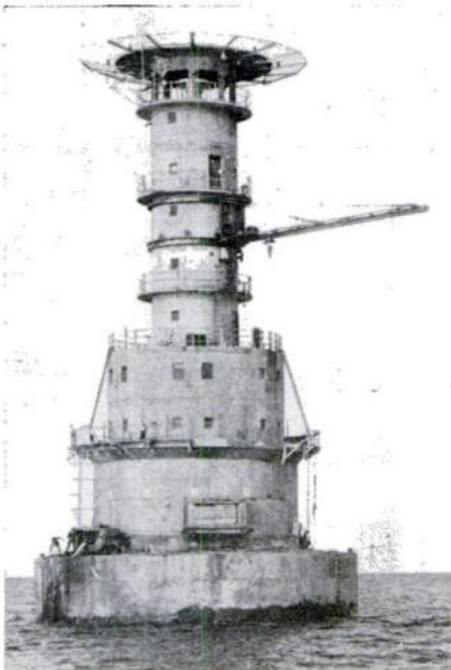
Transplanted lighthouse , built for the Irish by Danish engineers, rests in Dublin Bay. The unique lighthouse couldn't be built in the rough waters of the bay, so it was constructed in calm, shallow water, and floated out to the permanent site. There the foundation was sunk and secured, and the tower was raised and fixed in position.
