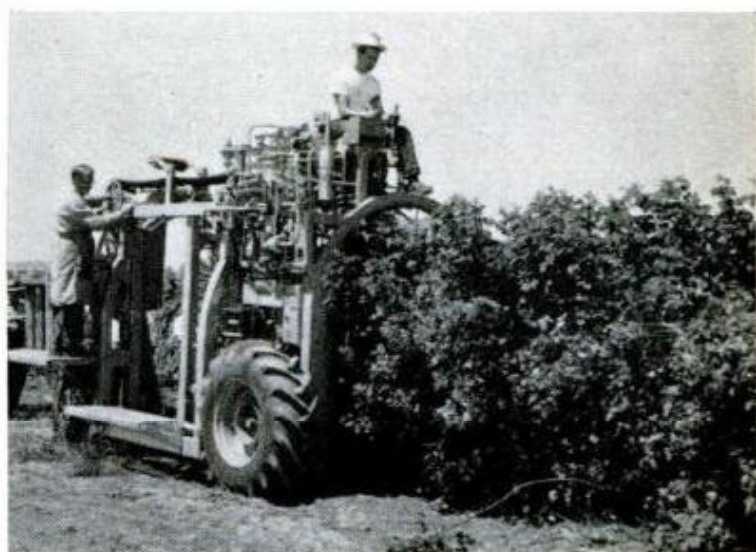
CANEBERRY PICKER uses hundreds of foot-long metal fingers on two freely rotating vertical drums to jar ripe berries loose from the plant. Berries then fall onto an endless belt
