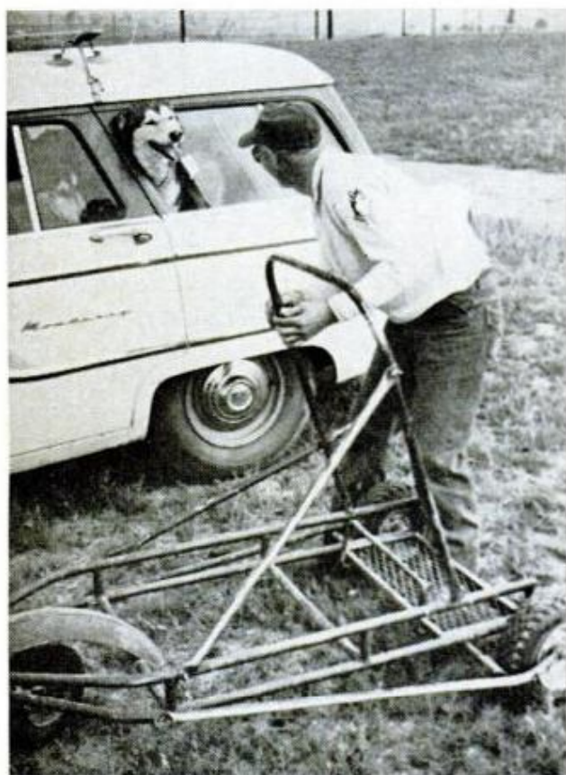
WHEELED SLEDS have not replaced the snow sled, and snow racing is still popular, but the three-wheel carts, which are little more than a steel frame with a steel mesh step for the driver, have enabled snow mushers to give added dimension to the sport
