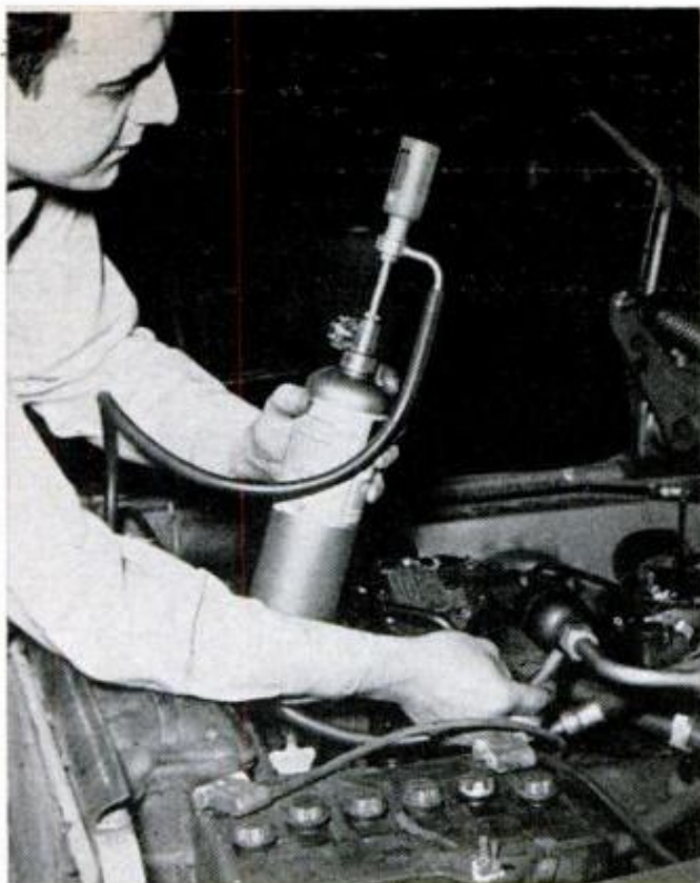
PROPANE TORCH DETECTS coolant leaks in the line and at connectors. Leaks cause flame to change color
