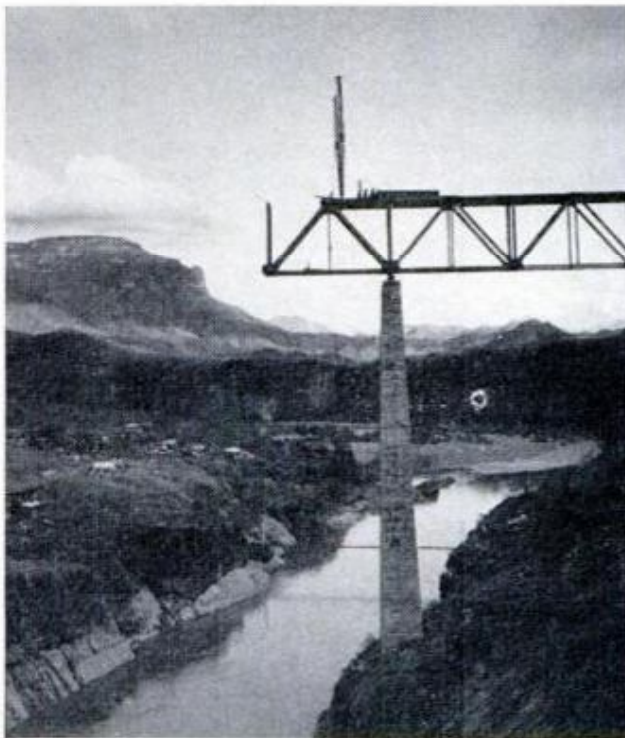
CONSTRUCTION HAZARDS included working on bridges as high as 350 feet up. This one, over Rio Fuerte, inches out from one concrete pilaster to the next
