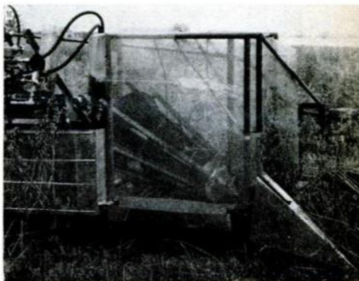
RICE THRESHER , developed for Southeast Asia, sends straw through rotor and concave; removes rice, starting at base of head, without cutting straw
