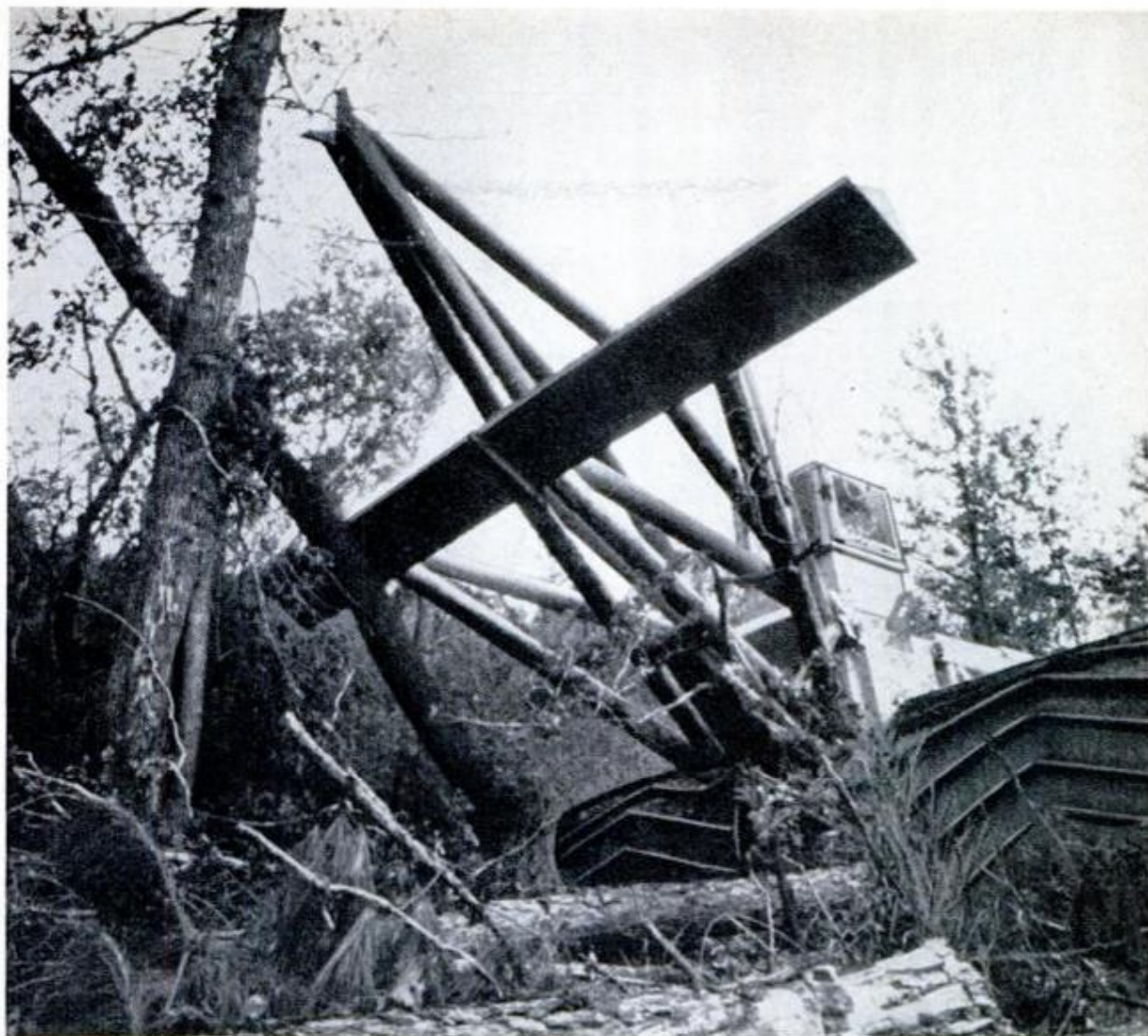
FORTY-TON BITE OF DIRT is scooped up in seconds by world's largest front-end loader (left) and dumped at the press of a button. Tree Crusher (above), newest LeTourneau machine, operates in swamp areas
