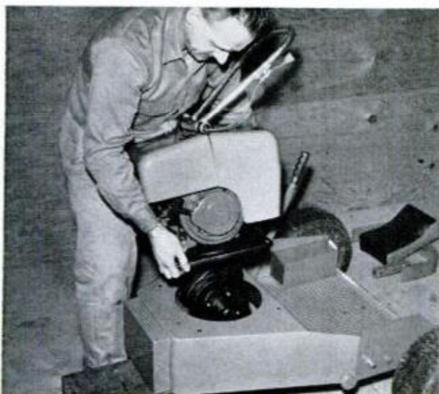
9. POWER WHEEL can be slipped into the body once the front has been propped slightly above level
