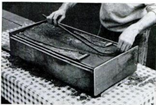
AFTER THE MOLD IS FILLED , press in the reinforcement at least 1 in. below the surface. Smooth over
