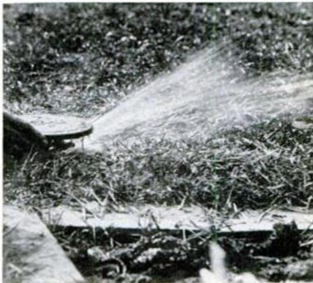
POP-UP HEADS are planted in holes 16 inches deep and held in place with coarse stone fill. When not in use, sprinkler head cover lies flush with ground
