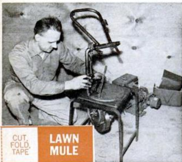
3. CLUTCH-BRAKE CAM and its control rod are installed next, followed by assembled control handle
