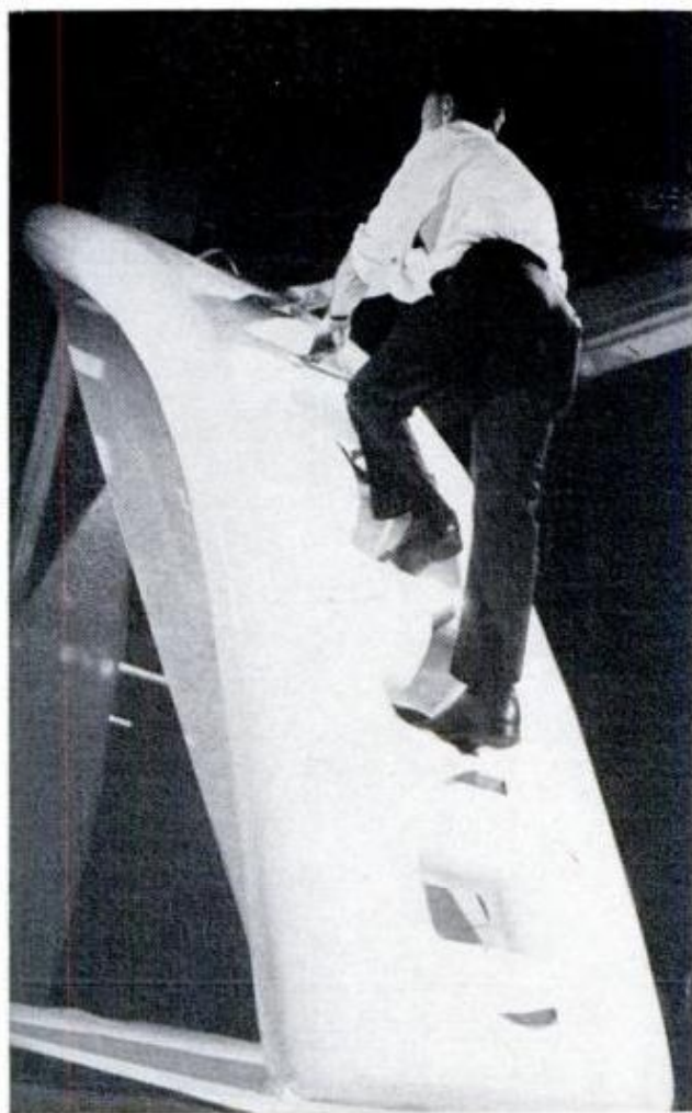
Air stair. Special inflatable ladders coated with white urethane rubber are used to inspect the insides of the Saturn missiles' rocket-fuel tanks, because ordinary ladders are too large to fit inside the 18-inch access ports. They can support two men.
