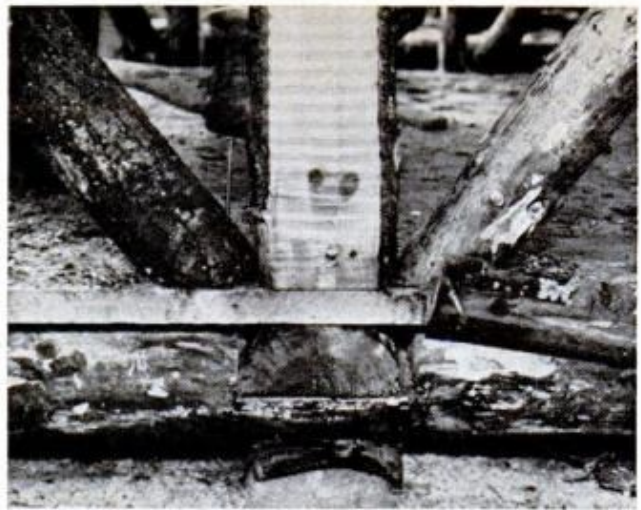
SPIKE the base of each cross brace to the floor slabs and spike the top to the upright posts. Cross braces should be as close as possible to the thickness of the trimmed upright posts
