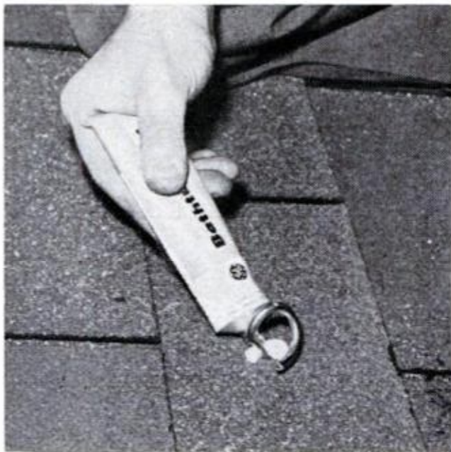
DAB OF SILICONE RUBBER seals holes around eye hooks. This is the easy way to prevent water leaks later. Takes only a moment, dries in about 12 hours
