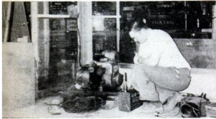
GENERATOR POWER turned fan to help dehumidify store. Dampness lingered long after flood had gone
