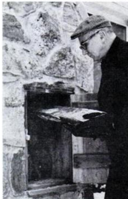
FIREPLACE INNOVATION is outside log-bin door permitting stocking wood in bin without hauling it through house
