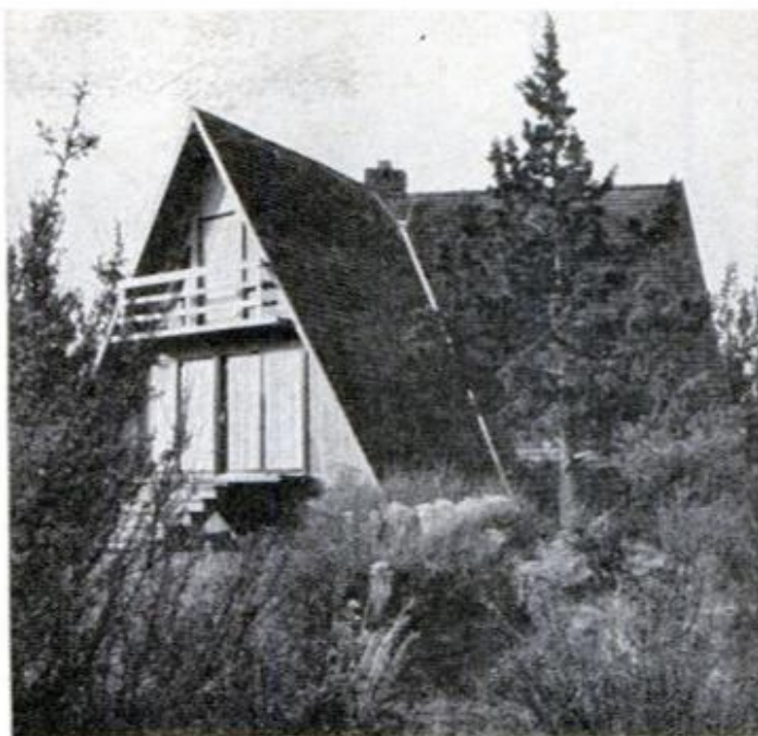
BLENDING WITH THE LANDSCAPE , the three-gabled A-frame is ideally suited to the rugged Northwest. The unique design offers 2500 sq. ft. of floor area on two floors
