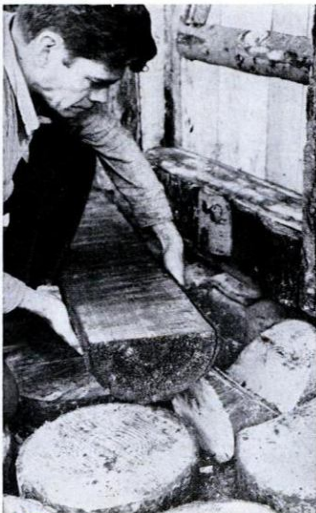
25. DOORSTEP is a 12-inch log, four feet long, ripped in half and set in notched blocks for footing. The 35 patio blocks are four-inch sections sliced from large log and set on ground as paving
