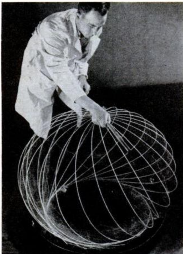
Expandable space antenna. No bigger than a briefcase when put into orbit, the antenna is said to be able to mushroom to a diameter of more than 60 feet. Made by Electro-Optical Systems, Pasadena, Calif., it's designed to reflect high-frequency signals. The antenna unfurls by means of the elastic energy created when its fiberglass frame is compressed.
