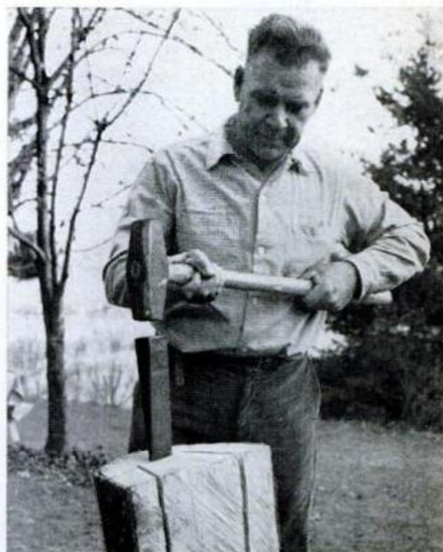
STEEL WEDGE , driven into base line of trough, chips out waste between kerfs. Pegged blocks close ends
