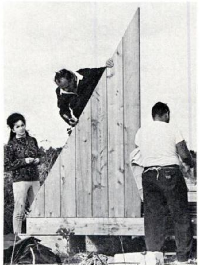
FOUNDATION BEAMS of 4x8-in. cedar or fir laminate are installed lengthwise on each of four rows of pilings. Owner Taughten (with pretty assistant) lends a hand nailing down flooring, while builder (left) prepares first module of front wall for assembly
