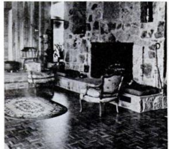
PATTERN COMBINATIONS with a tricky, new parquet flooring are possible with individual slats which can be removed at installation
