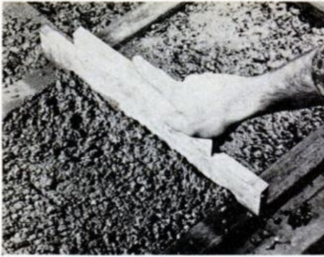
TECHNIQUE FOR A NEW FAD. One method for making colored blocks is given in text. Here's another: level concrete ½ in. from top of form; then add . . .
