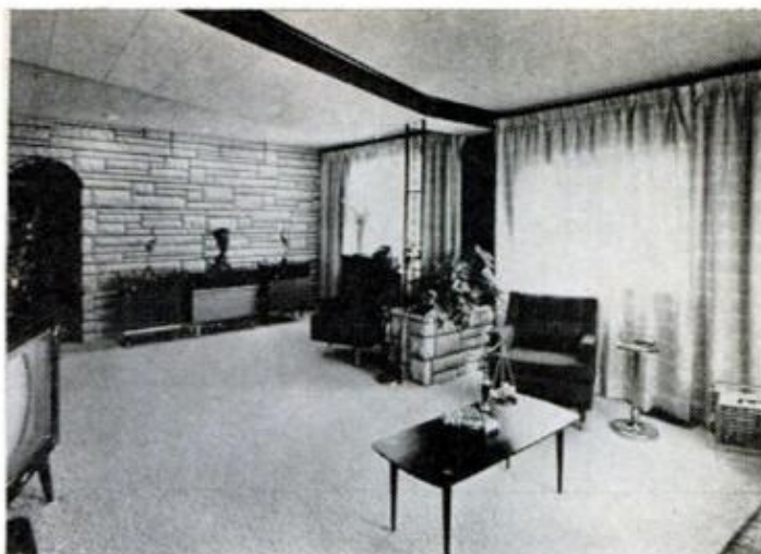
REALISM is achieved in panels by actually embedding crushed stone on the 12½ x 48½-in. surfaces. A finished accent wall of "stone" is example pictured above
