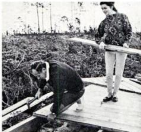
FOUNDATION BEAMS of 4x8-in. cedar or fir laminate are installed lengthwise on each of four rows of pilings. Owner Taughten (with pretty assistant) lends a hand nailing down flooring, while builder (left) prepares first module of front wall for assembly
