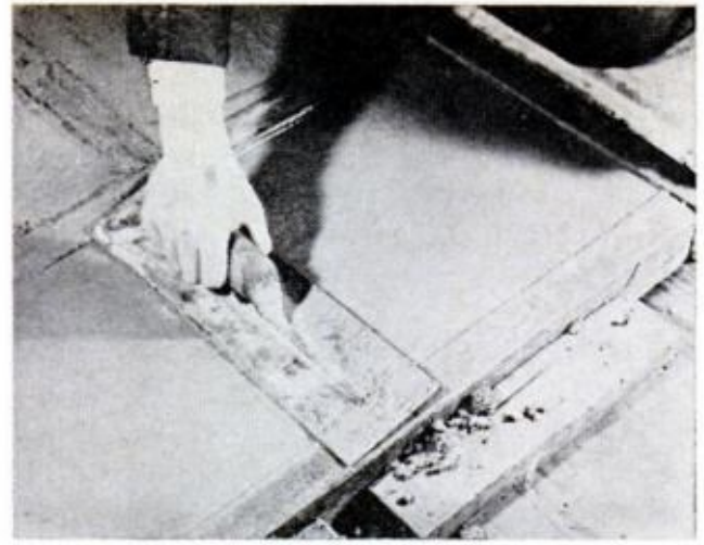
. . . TOPPING MIXTURE of 8 lbs. pigment, one 94-lb. bag of cement, 200 lbs. of sand, 5 gal. of water. Make a stiff mix and cast. Trowel and finish surface
