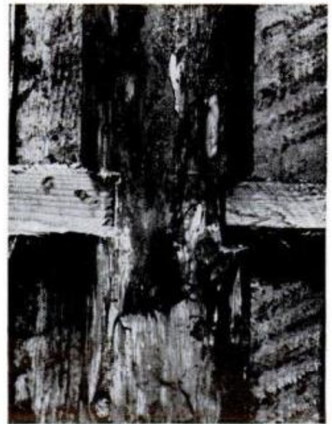
21. SIDING —much of it already on hand from squared-off logs—goes on vertically with 30d nails into cross framing. On front and rear walls, erect random lengths, then use chain saw to trim top ends
