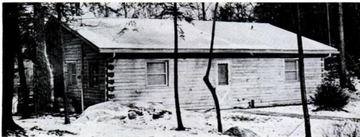
COMPLETED LOG CABIN measures 28x36 ft., with 15-ft. ceiling peak. All materials are precut, prefinished
