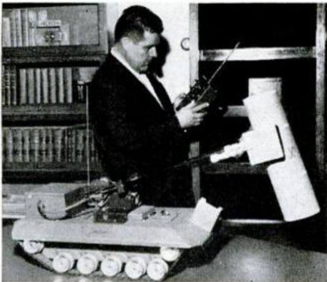
Bomb buster. No toy, this miniature tank is used by Montreal police to investigate and dispose of any potentially dangerous package by remote control while the operator keeps a safe distance. It can move up close, relay any ticking sounds to the operator's headset, take Polaroid pictures and return to the operator, or pick up the package and transport it to an unhabitated area for disposal. Wet-cell motorcycle batteries power the four motors—two to drive the vehicle and two to operate the arm mechanism.
