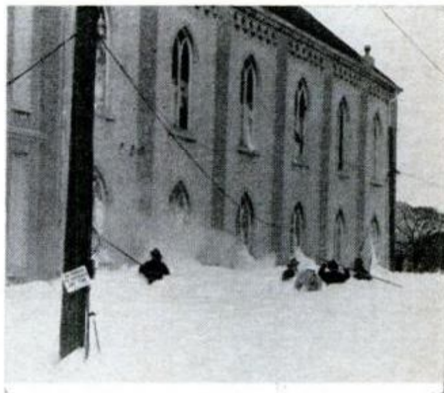
THEN CAME THE SUDS. Pumped into the church by means of a fabric tube, they soon filled the structure and poured from its windows, engulfing firemen
