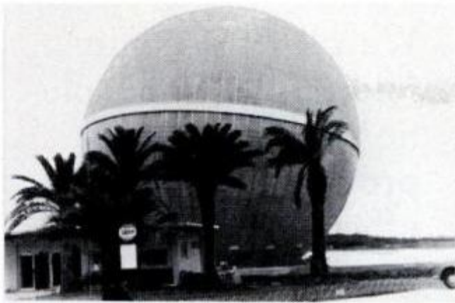
Floating globular greenhouse. In Ito, Japan, a 105-foot-diameter, steel-framed hot-house displays three floors of tropical plants and animals nonindigenous to the country. Located on a foundation in the middle of a pond and accessible only through a transparent, plastic tunnel, the greenhouse was built by the Totaku Izu Development Co.
