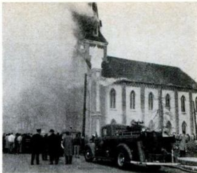
TOUGH TEST: Firemen in Dayton, Ohio, touched off the basement of this church scheduled to be razed, and allowed the fire to gain headway for 30 minutes
