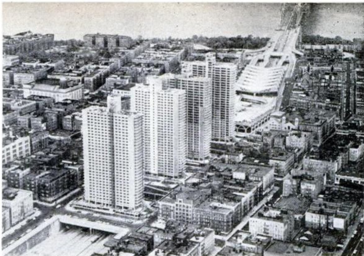
IN ALL, FOUR 32-STORY APARTMENT HOUSES and a bus terminal (behind them) straddle the 12-lane highway on the west side of New York City. Beyond the bridge is the New Jersey shore
