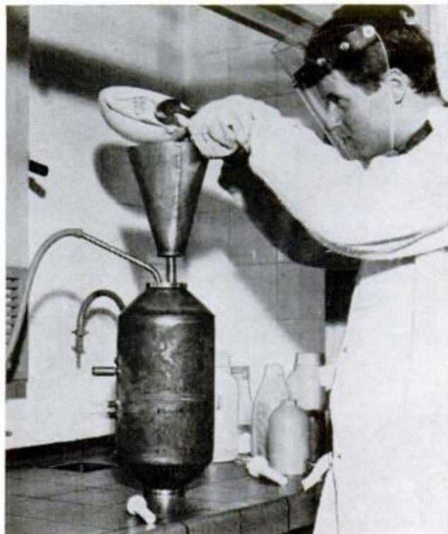
"COMET" IS MADE from simple steel barrel like this. It is being filled with chemicals that later will form its tail. The reactions are controlled at launch sites
