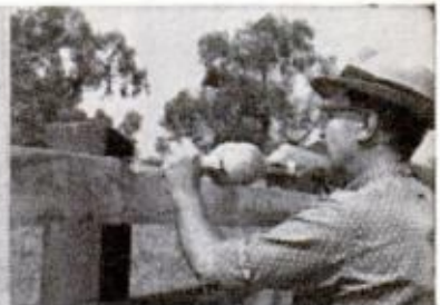
Trim fence posts
