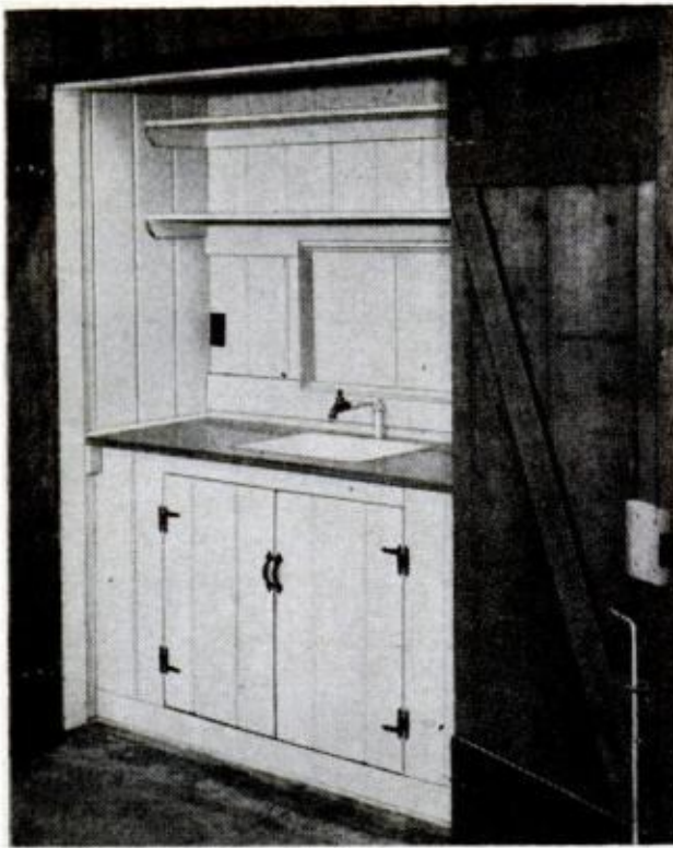
SINK ALCOVE , seen from patio (left), shows faucet, and duplex wall outlet left of pass-through. Back face of same wall (right) is paneled, has 1x12 shelves. Pass-through is handy when you need water inside garage
