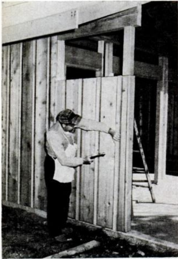
GAPS BETWEEN BOARDS needn't be uniform since battens hide them, but errors in alignment compound
