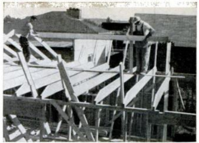
RIDGE POLE is installed in sections as rafters go up. Man at right is leveling ridge by means of marked upright—ridge pole will be nailed to it temporarily
