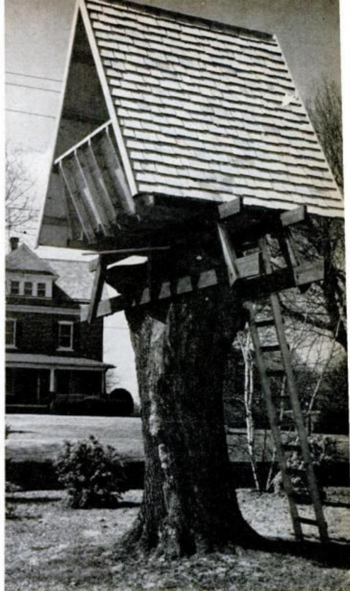
PERCHED ON STUMP of dead but solidly-rooted tree, this simpler A-frame needn't dodge branches. Built by Alfred Webber Jr., it sports red cedar shingles
