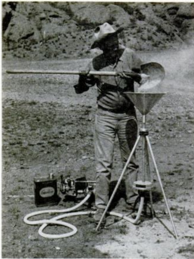
MIGHTY MIDAS is a dry concentrator. Pay dirt drops onto a small table where constant air flow and vibration separates the gold from lighter materials
