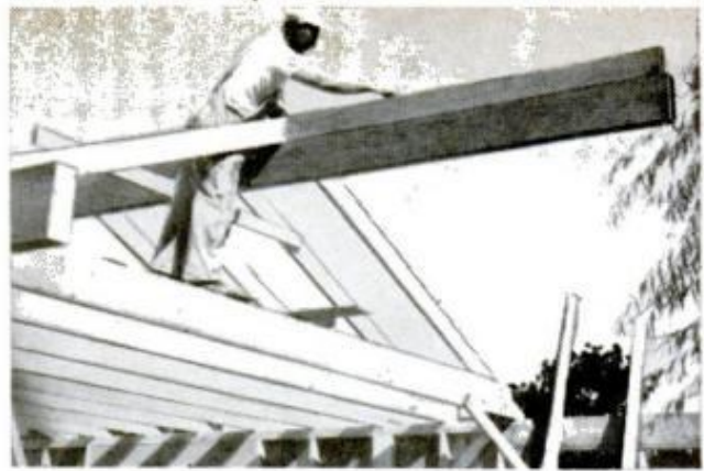
MORE RAFTERS are added, left—nailed to joists and to ridge pole (note temporary support at end)
