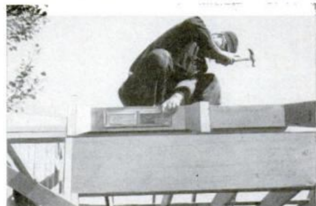
FRIEZE BOARDS are toenailed between rafters as shown in sketch left, photo below. Four are vented
