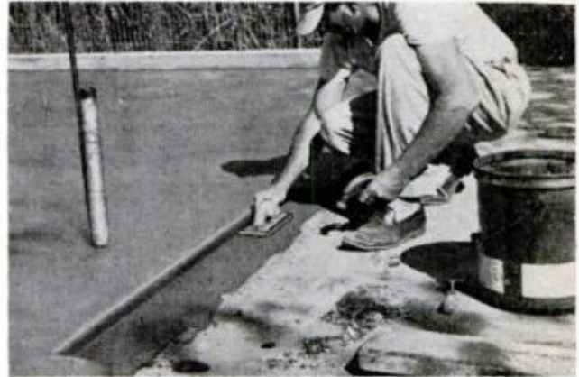
STEP-IN BAY at patio-edge of pour is finished off with rubber float, after removing cantilevered 2x6
