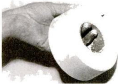
WHEN PATCH IS DRY, cover with joint cement, then apply two or three overlapping strips of joint tape
