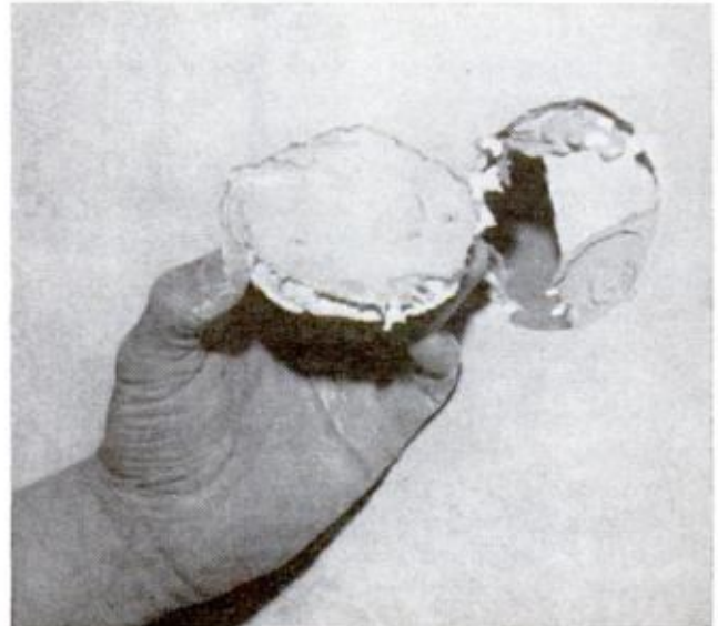
A FEW HOURS LATER , cement a plug of plasterboard to support piece and allow patch to dry thoroughly
