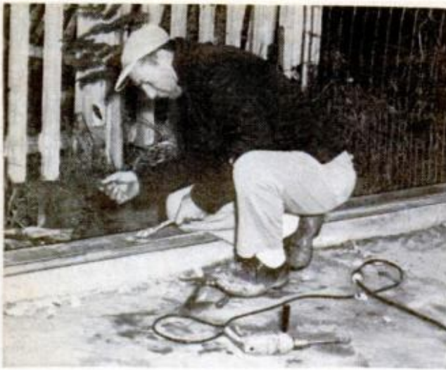
ANCHOR MUD SILL to top of foundation wall by drilling it to match protruding bolts, dropping it over them and turning the nuts up tight with a wrench
