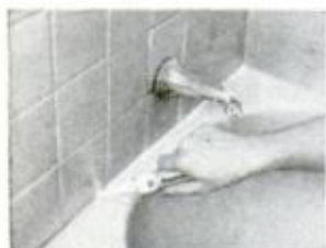
Caulk tub and tile
