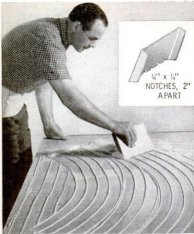
WHEN LAMINATING \frac{1}{4} or \frac{3}{8} -in. plasterboard over old plaster or plasterboard, spread joint cement on back of each panel with homemade tool (inset)
