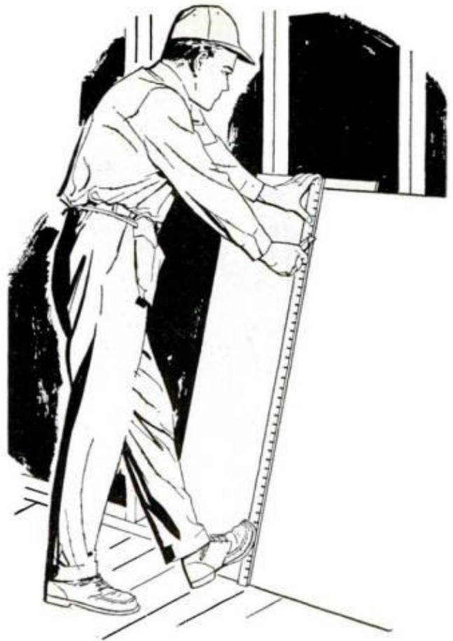
TO CUT A STRAIGHT LINE across the width of plasterboard panel (above), use a T-square to guide your knife. Drawing below shows undesirable bowing effect which is result of forcing panel into tight space
