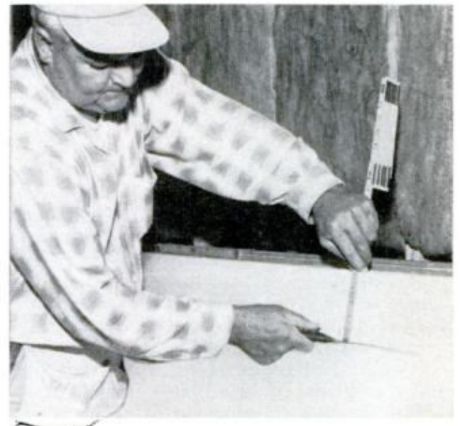
STRAIGHT LENGTHWISE CUTTING: Press your knife blade against the end of the ruler. Then, while applying enough pressure to score the plasterboard, guide the ruler along edge of the panel with your finger
