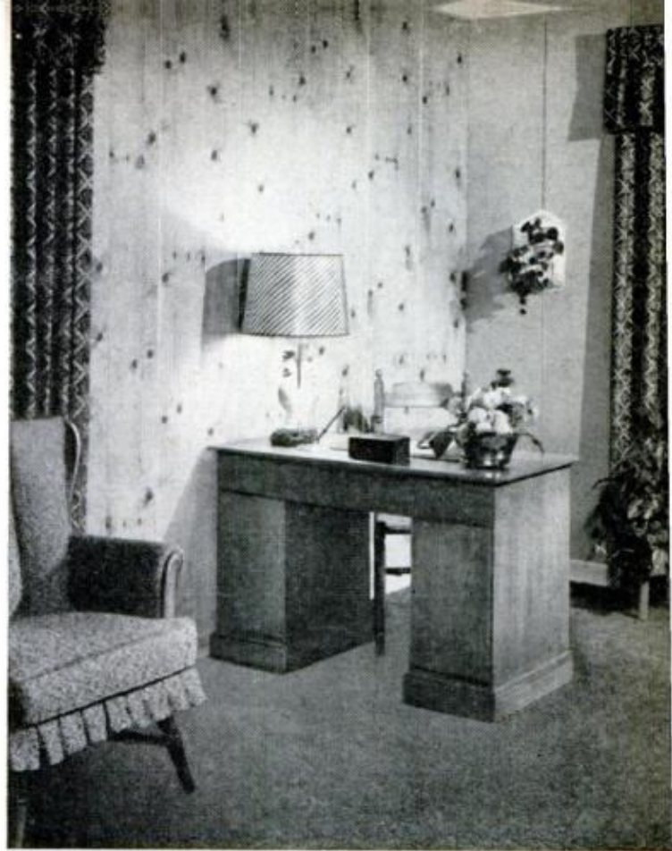
WITH PLASTERBOARD, amateur remodelers can obtain professional results. In room above, wall behind desk was "paneled" with wood-grain plasterboard
