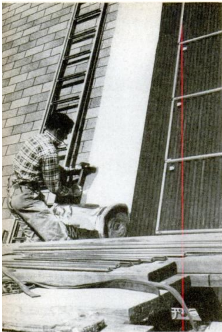
BUILDING heat trap on roof of newest house. Roof itself is insulated. On top goes layer of fiberglass, corrugated aluminum, topped by glass panes
