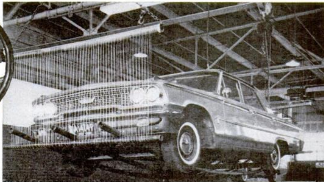
TWO-PLY TIRES USE bigger, stronger cord for similar total strengths as old four-plys. In demonstration photo (right), new cord carries total car weight
