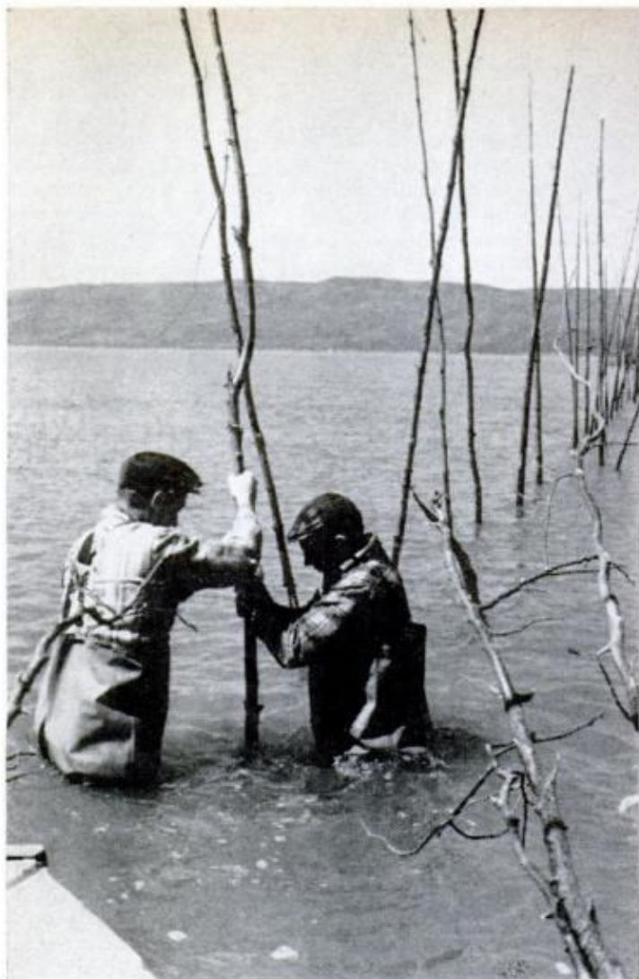
BUILDING THE FENCE for the weir, the whale trappers imbed saplings in the sandy river bottom. A strong current makes them shake, frightening a whale
