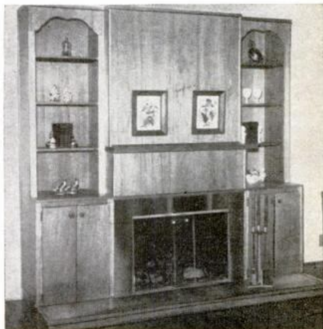
FIREPLACE prefabricated from hearth to chimney top installs anywhere. All-metal, 46 inches wide, unit needs no mortar, masonry or footings. Front opening model costs $300-350 installed. By Majestic Co., Erie St., Huntington, Ind.
