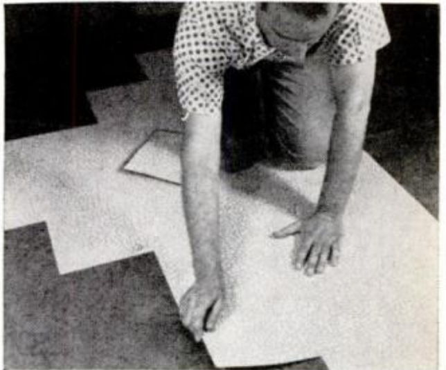
C. MARK BORDER TILE for cutting by laying a tile on last full row. Lay a second tile over it, butted against wall; mark first tile using second as straight edge
