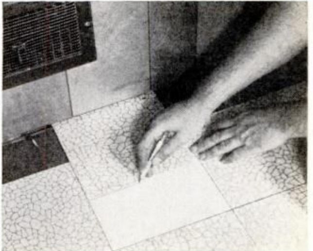
C. MARK BORDER TILE for cutting by laying a tile on last full row. Lay a second tile over it, butted against wall; mark first tile using second as straight edge
