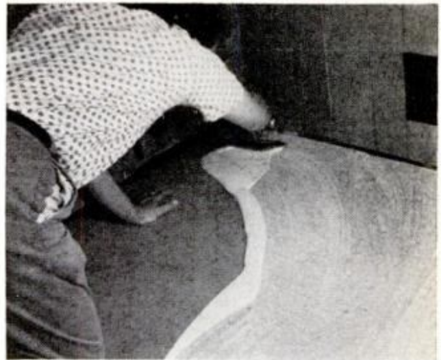
A. APPLY MASTIC over about half the floor. Be careful to spread it as thinly as possible, to minimize the possibility of adhesive coming up between the tile
