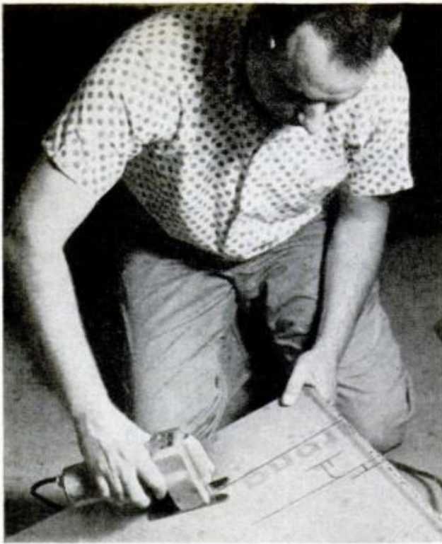
UNDERLAYMENT GRADE HARDBOARD cuts readily with standard power and hand saws. As shown above, a sabre or scroll saw is ideal for cutting the material to fit columns, corners, casings, and the like
