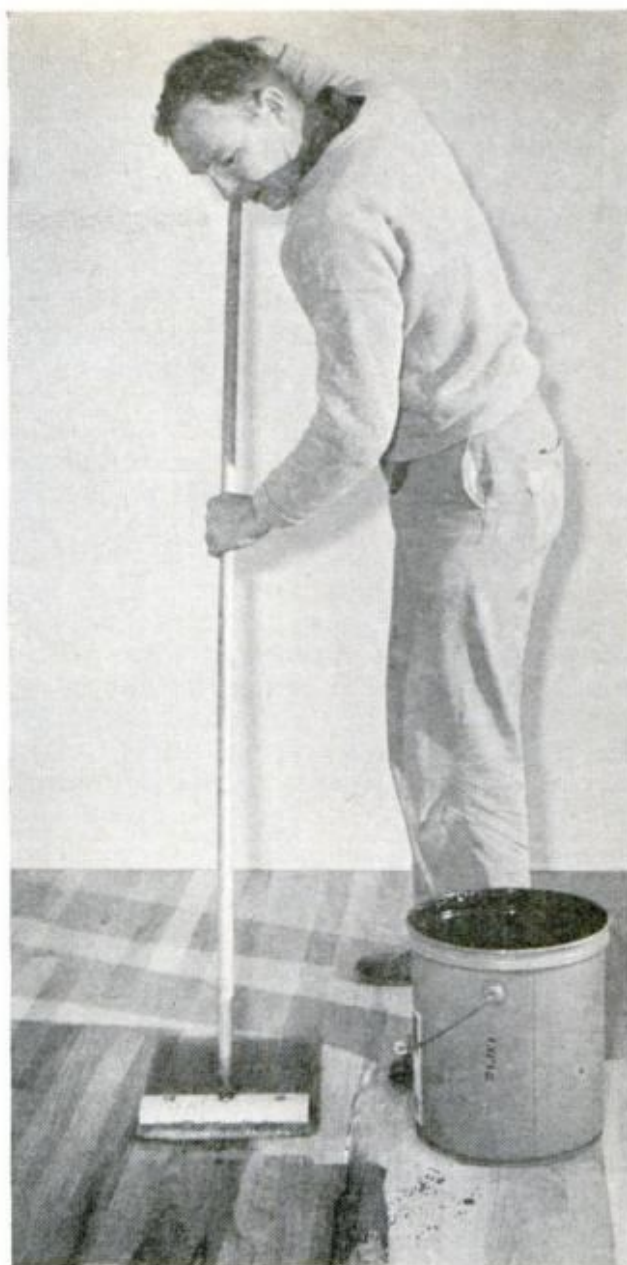
SPECIAL URETHANE floor finishes have extra abrasion resistance and last twice as long as varnishes
