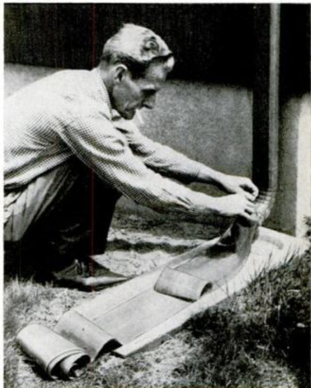
DOWNSPOUT SPILL , if not carried away from the foundation, may seep through basement walls. Plastic extension, below, carries rain water far from house, distributes it over lawn through sprinkler holes
