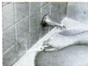
Caulk tub and tile
