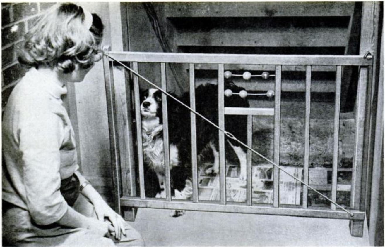
THE WASTE SPACE under a basement stairs can be put to good use as a pen for Fido. Plywood closes in the sides, and one side from a discarded child's playpen makes a gate when installed with hooks and eyes
