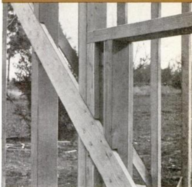
DIAGONAL BRACE is 1x4, set into notches cut across outer edge of studs (above). Notching in-place sole plate is difficult, so builders often recess 2x4 block between studs to anchor end of brace (below)
