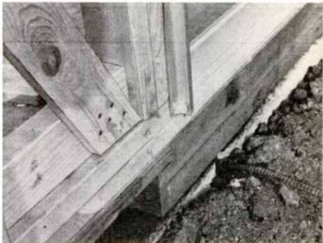
DIAGONAL BRACE is 1x4, set into notches cut across outer edge of studs (above). Notching in-place sole plate is difficult, so builders often recess 2x4 block between studs to anchor end of brace (below)
