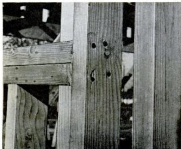
LOWER HALF OF SILL (to frame window opening) can be cut full width to slip between studs (above). Sill can then be nailed through outer face of outline stud as well as down into short studs beneath
