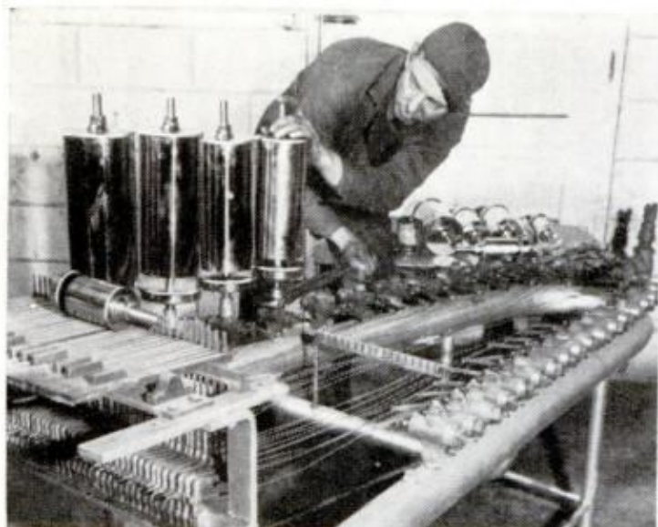
STEAM CALLIOPE , truly nostalgic sound of great old circus parades, receives new vocal chords. Originally built in 1903, it measures six feet in length
