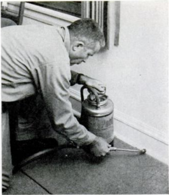
NESTS WITHIN WALLS can be treated by drilling ¼-in. holes every 16 in. along baseboard. Garden sprayer pumps liquid insecticide through these holes
