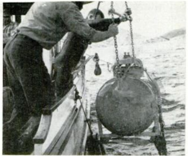
FILLED WITH FISH that normally live 150 feet below ocean's surface, the unique decompression chamber is lifted to the boat's deck by a mechanical winch
