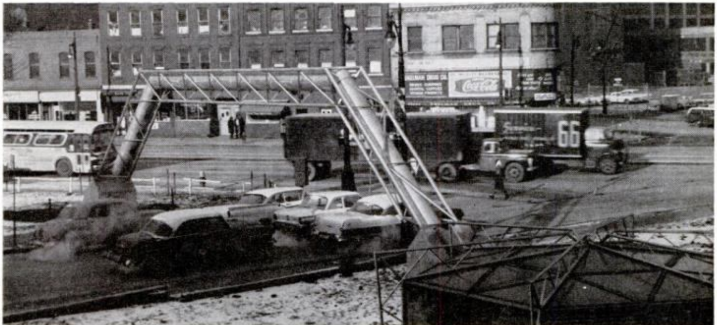
MAN'S TAMPERING with nature has thrown earth's CO 2 cycle (above) out of balance. A prime offender, researchers agree, is the automobile. Below, scientists at Wayne State University use this giant sampling machine to study auto's effect. Duct arches over Detroit street, draws in air for measurement of exhaust content
