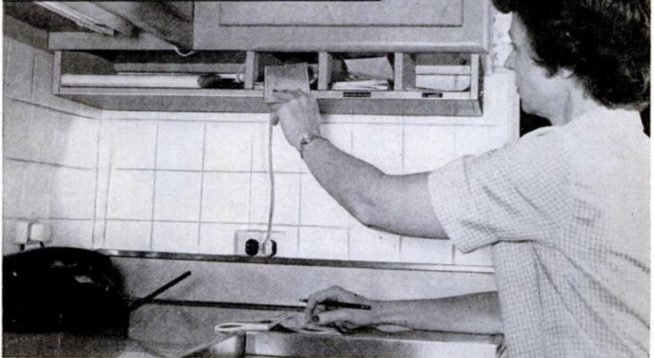
PIGEONHOLE RACK for mounting under hanging cabinet in the kitchen will turn the counter below into a kitchen desk. Make it from ½-in. plywood, as detailed above, and nail small facing strips over the exposed edges. Locate the partitions to provide separate compartments for telephone book, note pad, bills, unanswered correspondence, etc. To save trouble, paint unit to match cabinet before you bolt it in position
