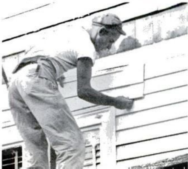
PLASTIC CLAPBOARD SIDING has stepped 8-in. face that makes it look like 4-in. boards. Inserts of fiberboard give extra stiffness and insulation value
