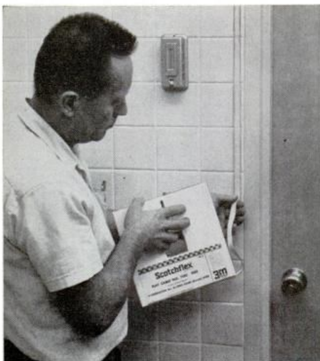
PROTECTIVE PAPER on cable's adhesive backing is removed before pressing cable in place. Available in gray or ivory, can also be painted to match wall
