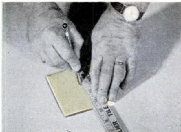
CUTTING TILE is a simple operation. Just score a line on the glazed surface with an ordinary glass cutter
