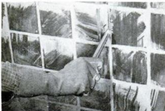
RAKE JOINTS with a striking tool. You can use any blunt-pointed stick—or even a toothbrush handle
