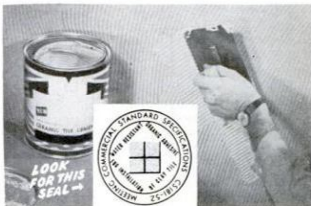
SPREAD MASTIC evenly over primed wall, using notched side of trowel so as to leave ridges in material
