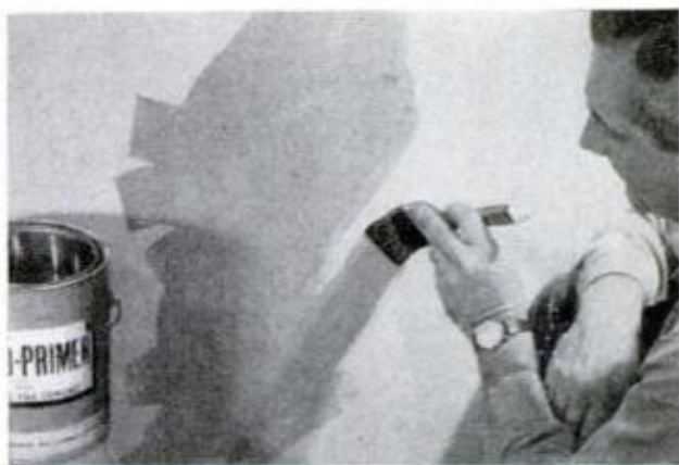
SPREAD MASTIC evenly over primed wall, using notched side of trowel so as to leave ridges in material
