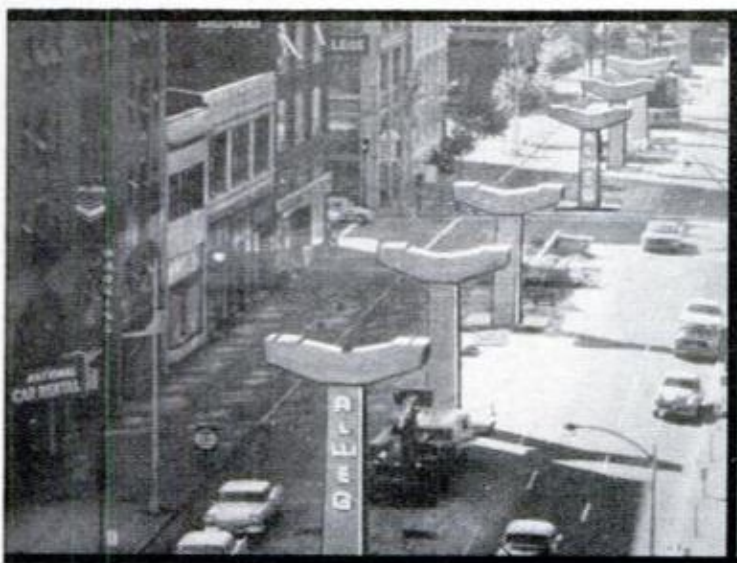
PRECAST CONCRETE COLUMNS of Alweg system hold both beams for two-way train traffic but still allow surface traffic to flow easily. Rail height is 25 feet
