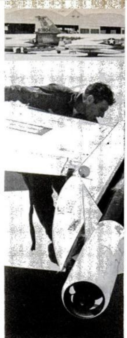
F-104 ARMAMENT includes bombs, rockets, missiles and cannon. Ground crew here hoists 750-pound bomb onto rack under one of its stubby wings
