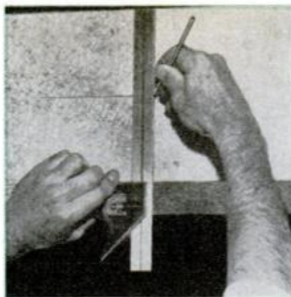
1. LOCATE center of duct where zoning damper is to be installed
