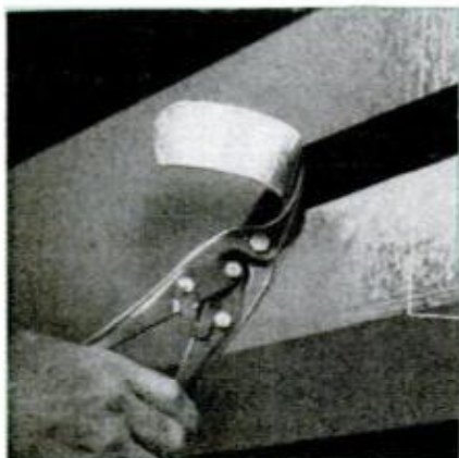
6. CUT slot in front of duct so that damper blade may be inserted
