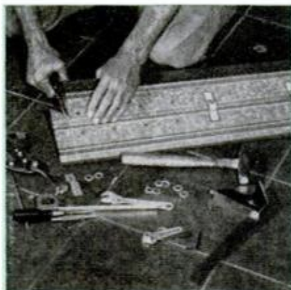
7. TRIM blade to match duct width, allowing \frac{1}{8} -in. clearance at ends
