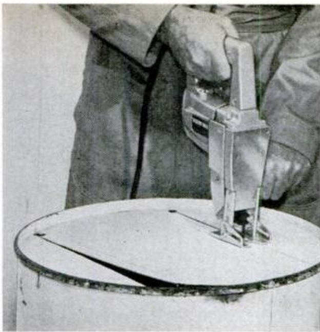
ASH-DUMPING DOORS fit into a 10-in.-wide opening sawed out of the bottom of the 30-gal. drum. Orient cutout so drum seam will be at the rear of burner
