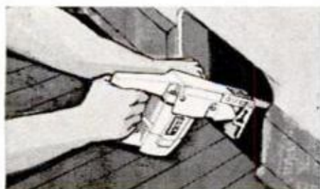
Cuts in Walls, Floors
