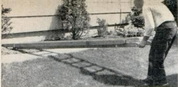
1. Working alone? No problem, if you butt the foot of the ladder against the wall, then lift other end
