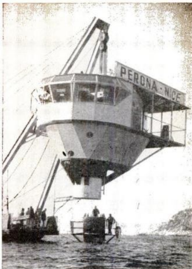
LOWERED INTO PLACE to cap the 180-foot tube, this floating island will house scientists studying the habits of sea life from within the submerged tube
