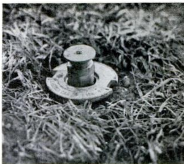
POP-UP SPRAY HEAD comes up about 1 in. when water is turned on, enabling spray to clear nearby grass
