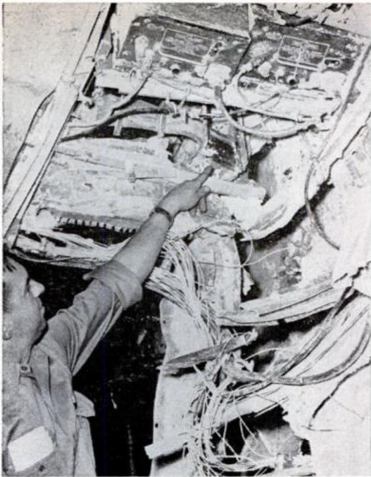
SOME RECORDERS are carried in plane's wheel well, others in radio rack. Employee points to niche which carried recorder of F-27 that crashed in Salt Lake
