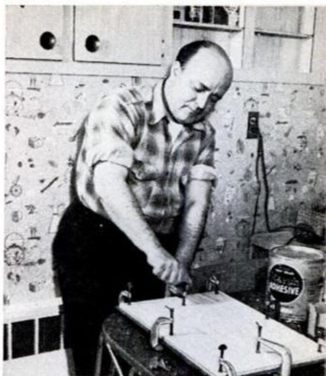
BOND DOOR FACING to plywood so it projects equally on all sides; this forms a \frac{3}{8} -in. lip that overlaps the opening, as shown below. A 25-deg. chamfer dresses up the edge. Apply C-clamps or weights
