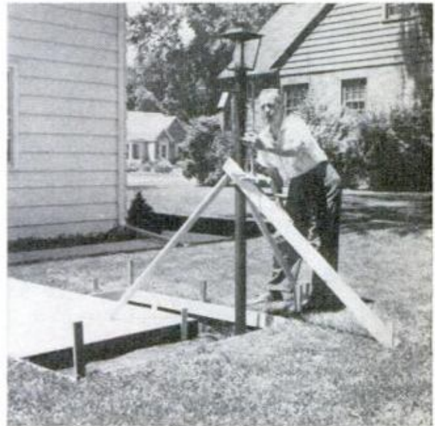
POST IS CHECKED (above) to be sure it's plumb prior to pouring footing. I used a couple of C-clamps to clamp the braces to the post. Below, form has been filled and I'm smoothing it off. It required about half a yard of ready-mix, will vary with footing depth
