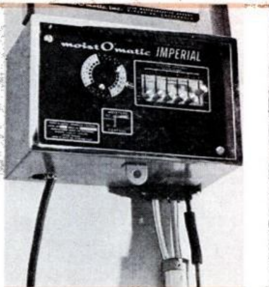
HYDRAULIC CONTROL unit can be mounted on any wall, inside or out. Metal pipe protects plastic tubing
