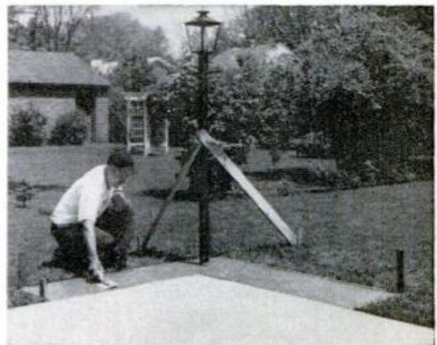
POST IS CHECKED (above) to be sure it's plumb prior to pouring footing. I used a couple of C-clamps to clamp the braces to the post. Below, form has been filled and I'm smoothing it off. It required about half a yard of ready-mix, will vary with footing depth
