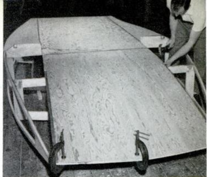
AFTER SECURING aft edge of bottom bow planking, clamp fore end to bow beam and add other fastenings. Outside bow planking notches to center section
