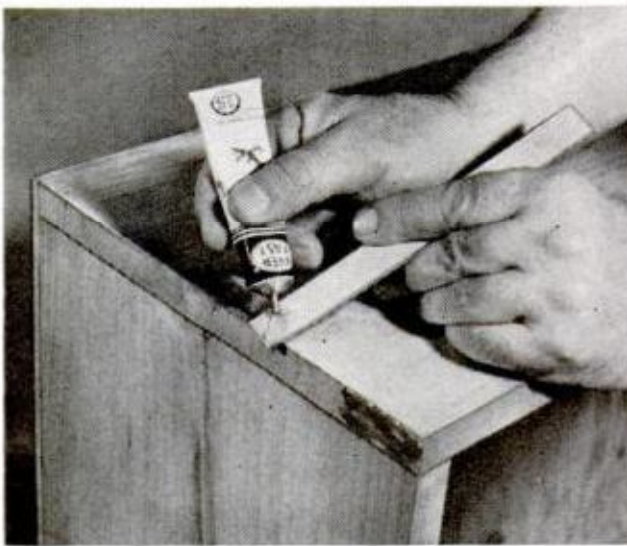
2. TO SEAL END GRAIN , try applying a thin coat of cellulose cement with a spatula, then scraping off excess. It dries in a hurry and is a real timesaver
