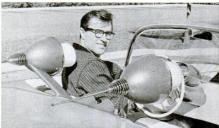
FRONT OF CAR sports three pairs of running lights in all. Futuristic headrests house radio speakers, protect against whiplash
