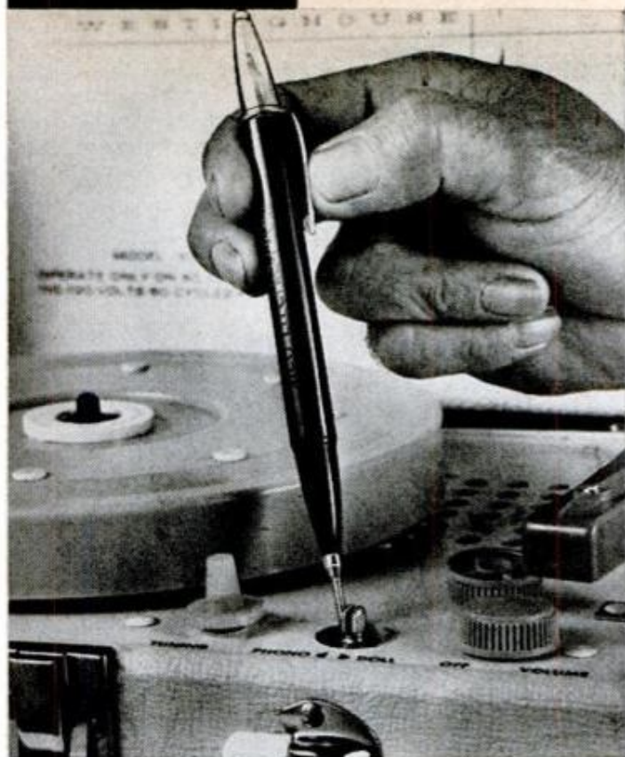
SHOCK CHECKING phonograph chassis (upper left) and heat testing toy vegetable (upper right) with temperature-indicating paints—two of the tests which supplemented an expert judging of the PM toys' play value
