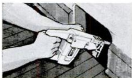
Cuts in Walls, Floors
