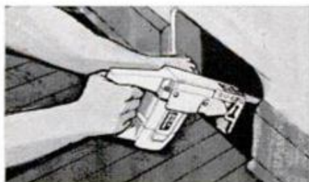
Cuts in Walls, Floors
