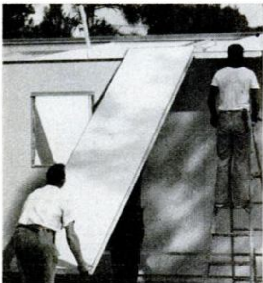
ALUMINUM PANELS are easily slid into place by one or two men. Panel joint (below) slides down to lock both crimped edges of each panel
