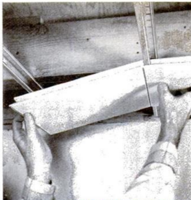
TONGUE-AND-GROOVE joint between tiles conceals the flange of metal Z-strip from which ceiling is hung
