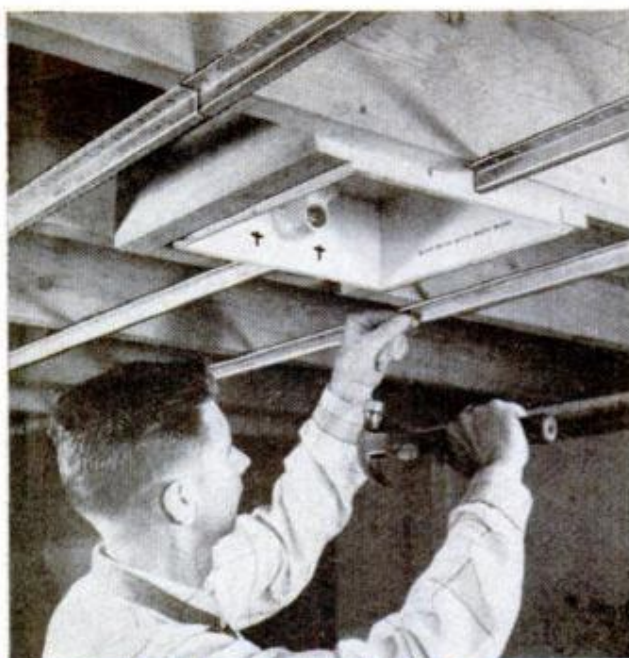
INSTALLATION of lightweight metal furring strips is much easier than nailing ordinary wood furring
