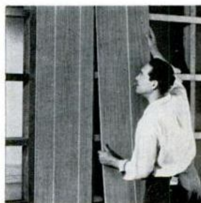
Tongued-and-grooved Marlite Random Plank (16" x 8" x 1/4") goes up fast over furring strips or solid backing with no waste, muss or fuss.
