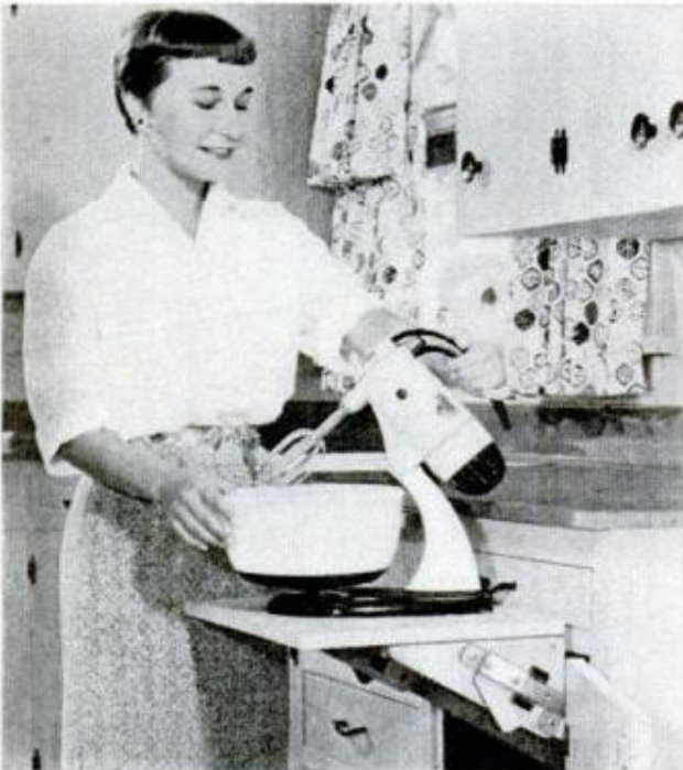
APPLIANCE SHELF operates just like typewriter shelf that closes into desk. Shelf folds into cabinet below
