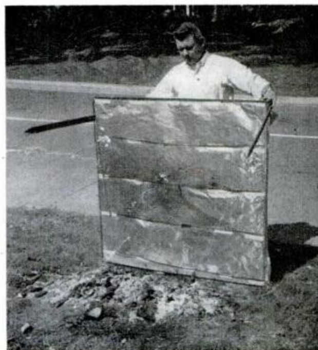
REFLECTOR SHIELD made of aluminum foil tacked over a light frame will hasten the burning of a stump
