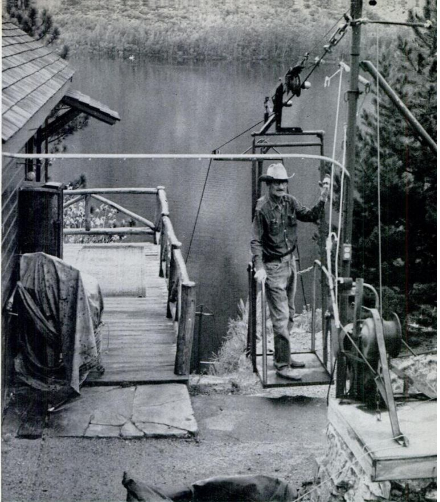
HILL-CLIMBING tramway saves a 50-foot climb by hauling people and boats from this cottage to the lake
