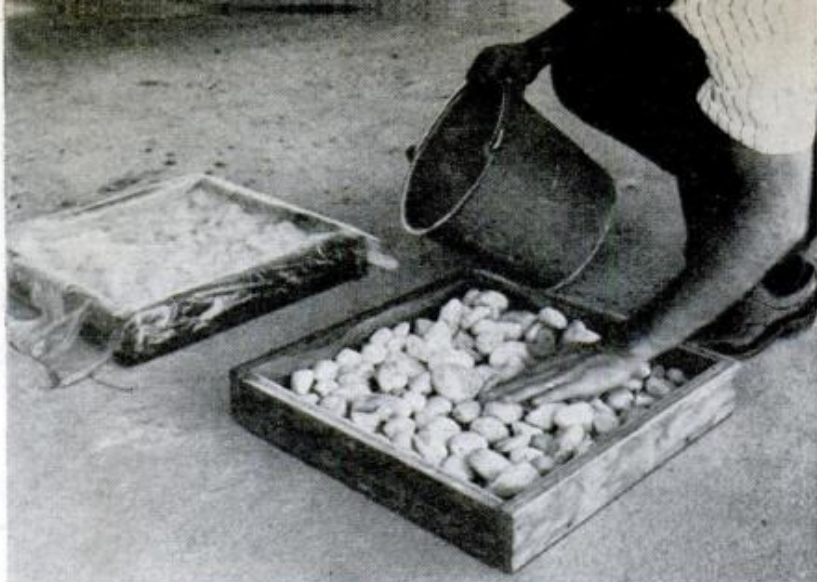
CASTINGS made in this fashion can be used as flagstones or, with a little ingenuity and imagination, they can be used as pattern insets in a retaining wall of blocks or other masonry
