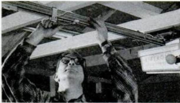
BLACK TUBE (above) curtains ambient light. (Below) limit switches are installed on guide rails of door
