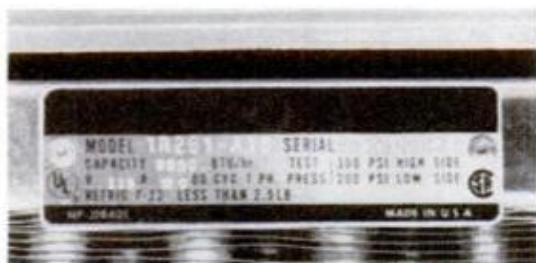
BTU RATING should be stamped on unit; if it isn't, see manufacturer's specification sheet
