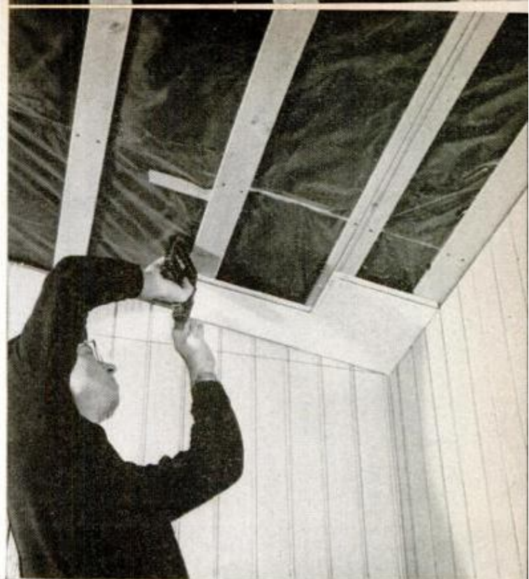
BORDER TILE at ends of every other row are cut in half when joints of tile are staggered. Initial starting tile in very corner measures 10 x 12 in.
