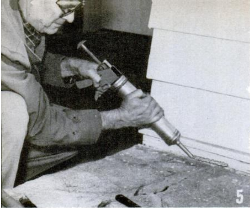
6 SEALING OPEN JOINTS IN SIDING
