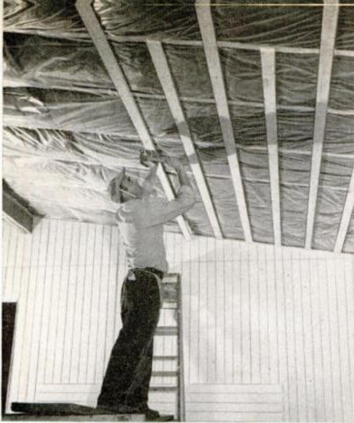
FURRING STRIPS nailed directly to edges of rafters and spaced 12 in. on centers, are required to provide stapling surface for 12-in. fiberboard tile
