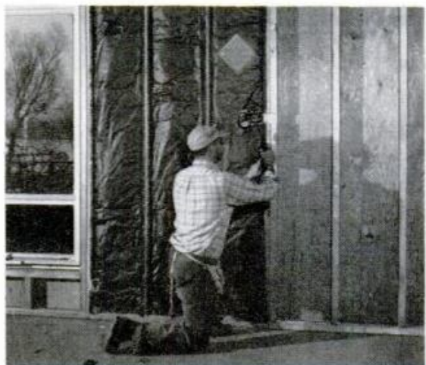
WHEN WIRING is in place in exterior walls, blanket insulation is installed and stapled to the studs
