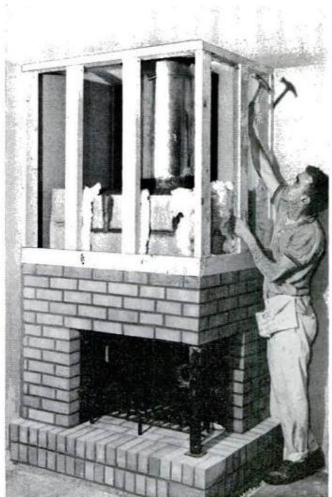
FINISHED FIREPLACE , with masonry and paneling concealing prefab, passes easily for original equipment WITH FOUNDATION laid through basement, base form goes in place, below left. Right, frame for paneling
