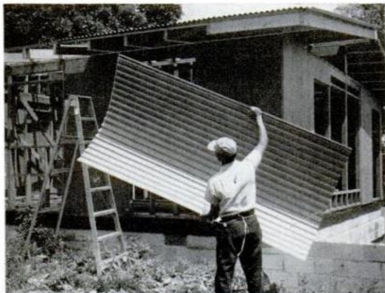
PILOT HOME has roof of colorful corrugated aluminum supported by 2 x 4 purlins nailed to rafters and spaced approx. 24 in. apart
