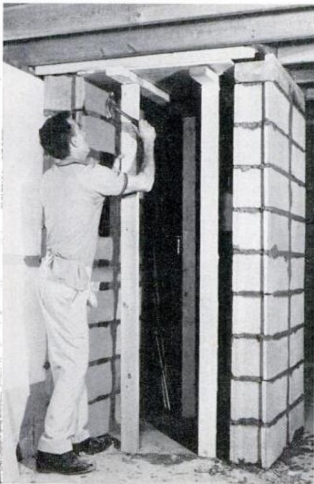
FINISHED FIREPLACE , with masonry and paneling concealing prefab, passes easily for original equipment WITH FOUNDATION laid through basement, base form goes in place, below left. Right, frame for paneling
