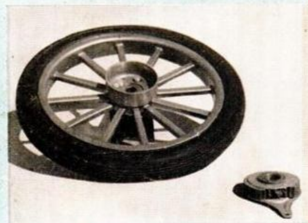
3. BRAKE DRUM bolts to inside of left rear wheel, and brake shoe assembly is mounted on the axle itself
