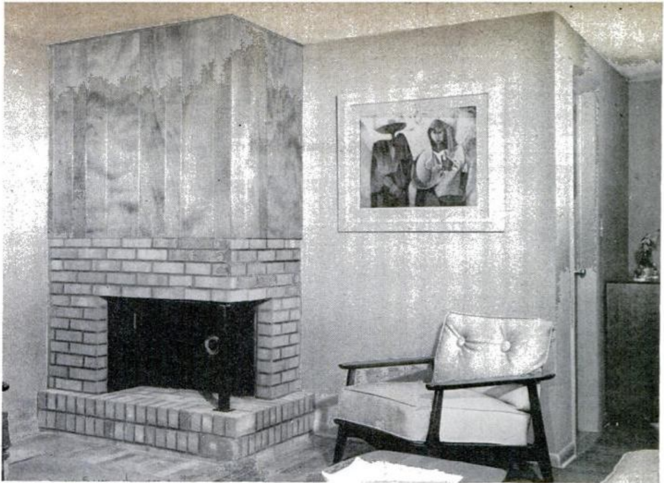
FINISHED FIREPLACE , with masonry and paneling concealing prefab, passes easily for original equipment WITH FOUNDATION laid through basement, base form goes in place, below left. Right, frame for paneling
