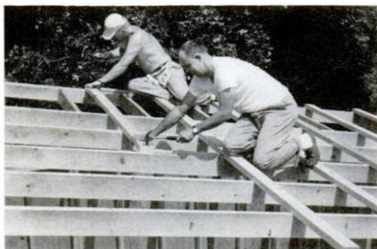
PILOT HOME has roof of colorful corrugated aluminum supported by 2 x 4 purlins nailed to rafters and spaced approx. 24 in. apart
