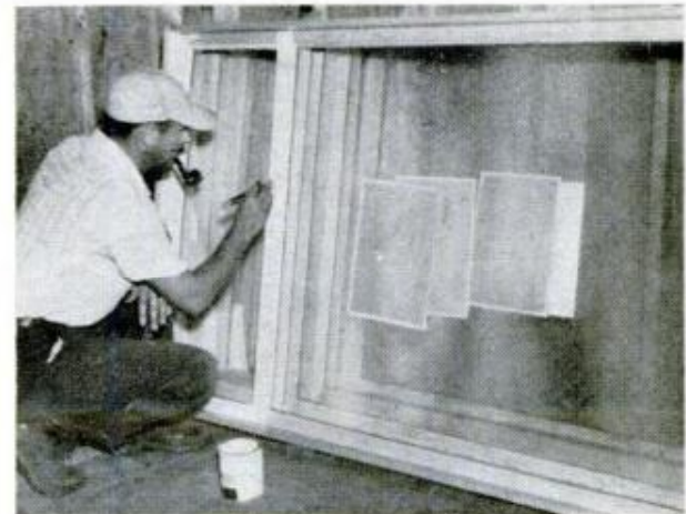
C-CLAMPS ARE USED to hold wall sections in line while spiking abutting studs together, above. Time can be saved on the job by priming window and door frames at home before carting them to building site
