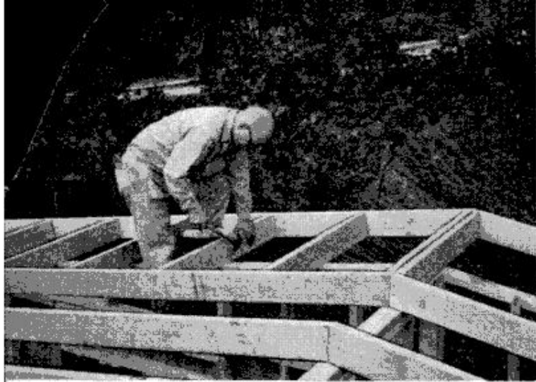
RAKE PANELS which form the overhang at gable ends of roof are toenailed to the supporting gable plate
