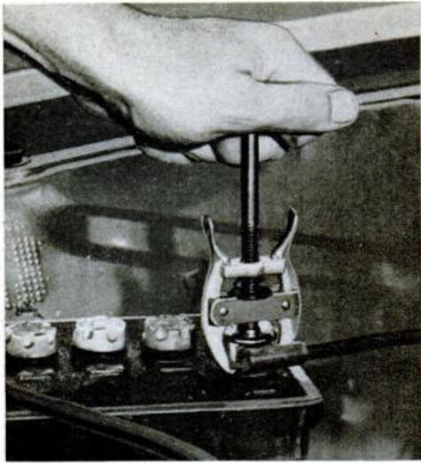
11. BATTERY-CLAMP PULLER removes the cable clamp from the post without damage to the post or clamp
