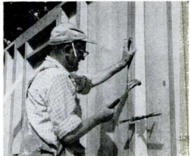
C-CLAMPS ARE USED to hold wall sections in line while spiking abutting studs together, above. Time can be saved on the job by priming window and door frames at home before carting them to building site
