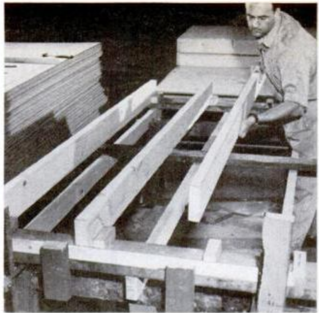
STOP BLOCKS automatically position longitudinal members in nailing jig in fast assembly-line operation
