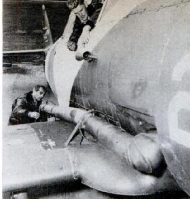
SKY SMOKE is discharged from specially designed tube mounted along fuselage of each plane in group
