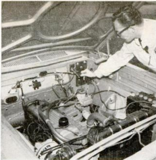
BULKHEAD WIRING CONNECTOR —a good idea, but PM test car's horn wire and starter lead each loosened
