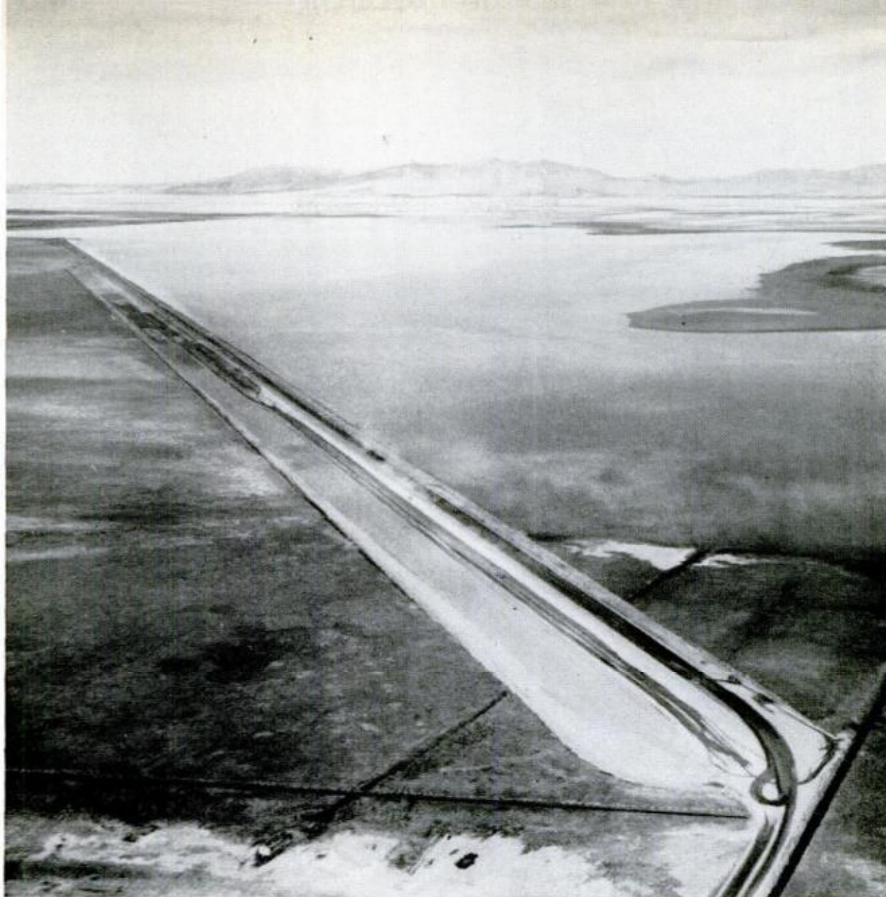
WILLARD DAM will have dual purpose, keeping out salt water from Salt Lake (right) and impounding fresh water in basin now under construction (left). Aerial view shows north portion of dam which will be 12 miles long
