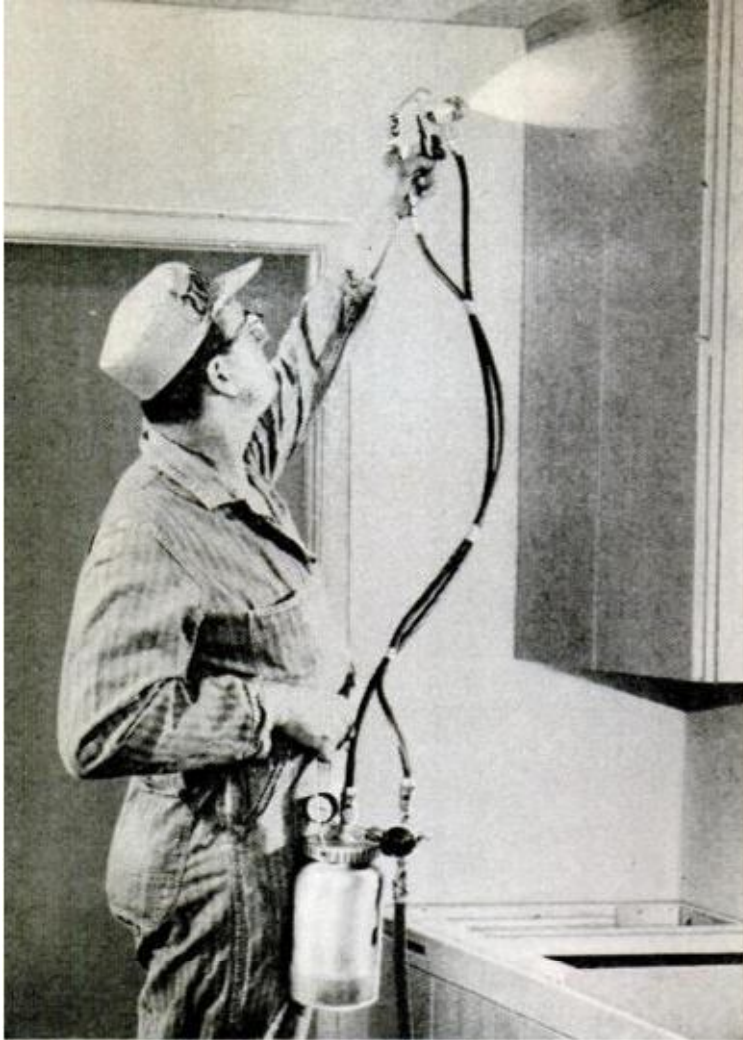
8. THIS SPRAY UNIT has a portable paint cup, or container. Unit is operated on an air line from a compressor. Gun and container are small and readily carried from room to room or job to job as needed
